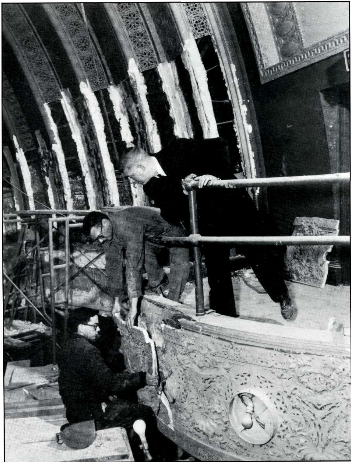
John Vinci (seated), Richard Nickel (left), and John Dienhart of Field Enterprises, which provided funding for architectural salvage at the Garrick, remove plaster panels from the inside of the theater.
