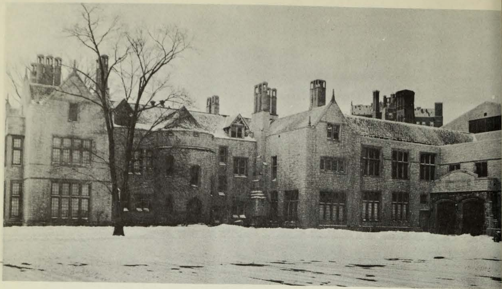
Side-view of the Rand Mansion with the adjoining Consistory
