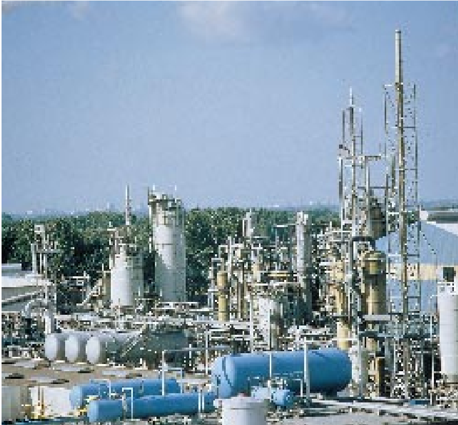
The Kemira Pigments titanium dioxide plant in Rotterdam is increasing its capacity by eliminating bottlenecks. The nickel removal plant that is soon to be built will further purify effluents from the plant.
