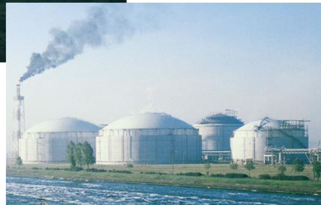
The fuel reservoirs at the Antwerp harbour depot are built from Rautaruukki's installation-ready prefabricated steel plate.
