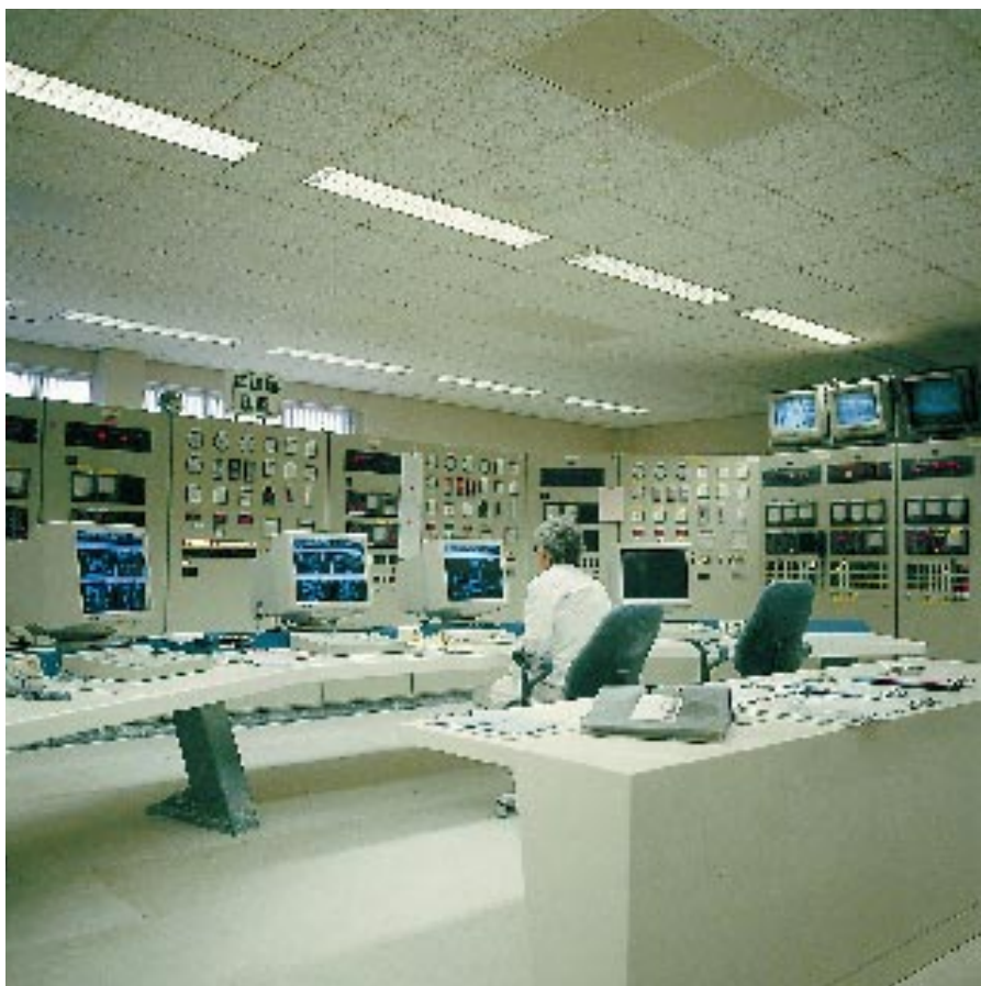
The production of the Rotterdam plant was modernized in order to expand the product range and thereby the customer base.
