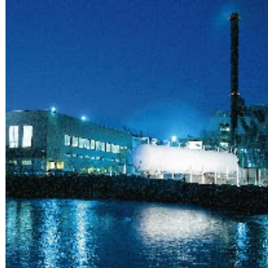
Tehokaasu Oy retained its market position in deliveries to industry.
