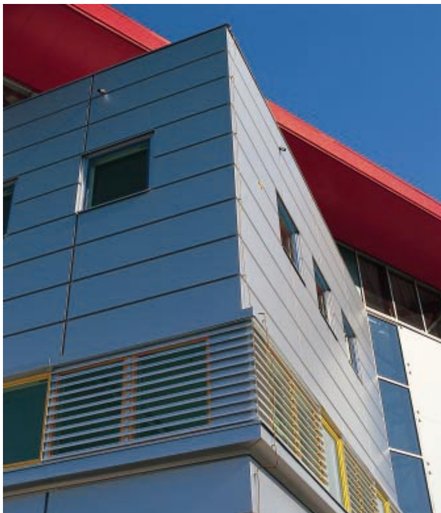
Bright new colourant factories were completed for Tikkurila CPS in Australia, the United States and Finland (in the picture) in 1997. (Photograph: Peter Forsgård)
