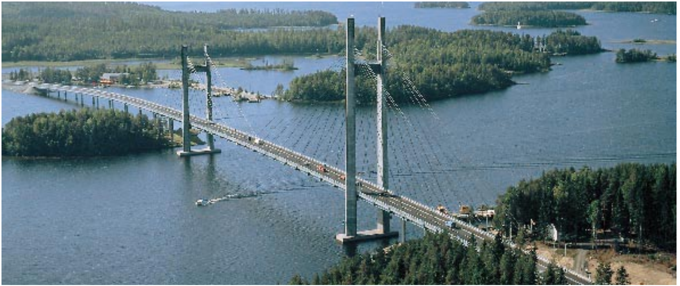
The Kärkistensalmi Bridge in Korpilahti, Finland, which became operational in August, is protected by Tikkurila anticorrosion paints. (Photograph: Lentokuva Vallas Oy)
