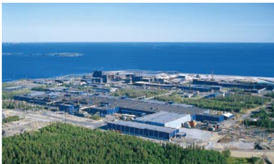
Outokumpu owns a 250-hectare land area at Röyttä in Tornio. About 10 % of the area is currently covered by buildings.
