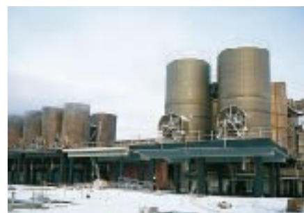
The expansion of the Kokkola zinc plant in Finland has progressed according to plan, and zinc production has proceeded at normal levels at all times. Pictured are new cooling columns.
