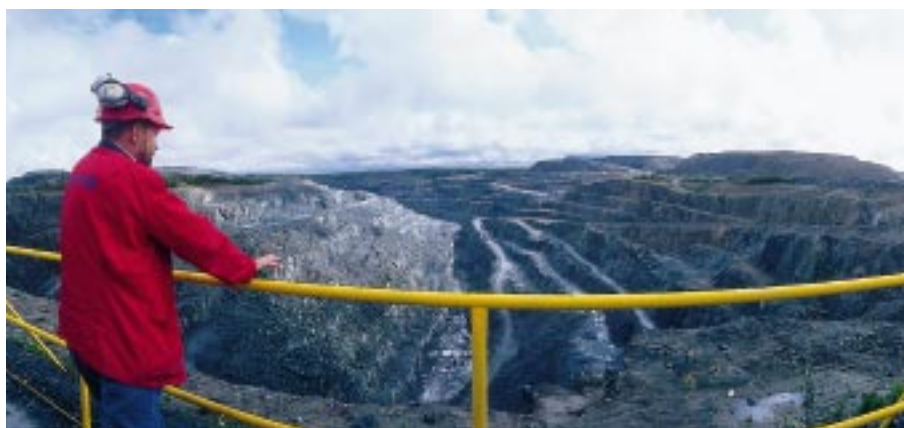
The Kemi open pit will convert to underground mining. The project started in the beginning of 1999 and is estimated to last for five years. Ore mined in 1998 amounted to one million tonnes.
