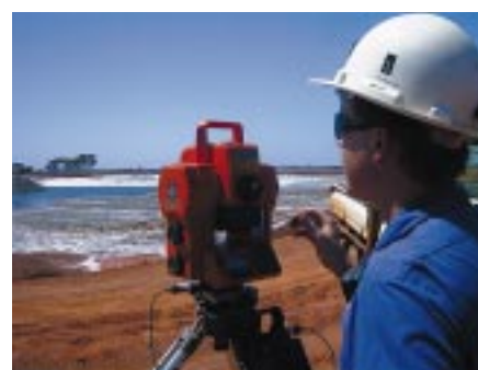
Surveyor Myles Ertzen completing leveling work at the tailings area of the Black Swan nickel mine (previously Silver Swan) in Western Australia. Since the beginning of November, the mine is wholly-owned by Outokumpu.
