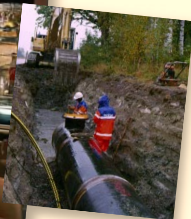
A main water pipe supplied by Metform being laid in Norway.
