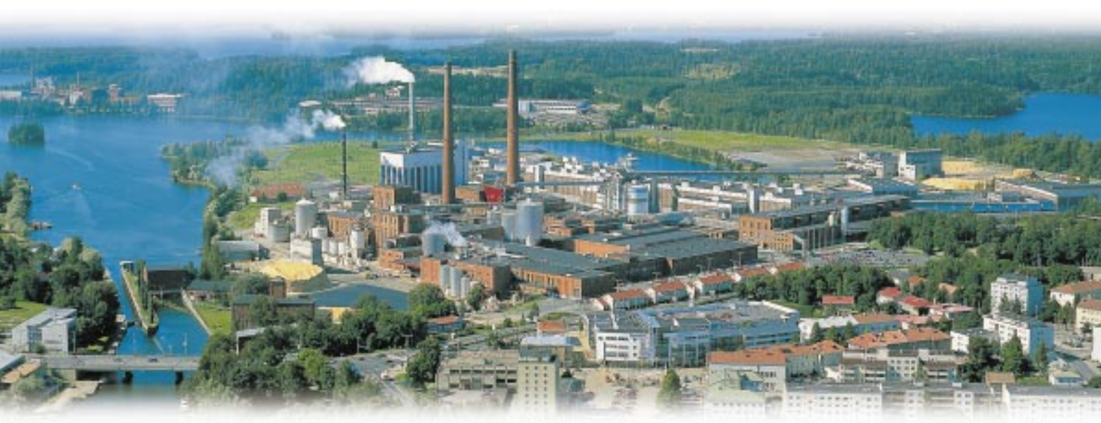
Residential areas have sprung up around several of UPM-Kymmene's mills. Pictured here are the Tervasaari pulp and paper mills in Valkeakoski.
