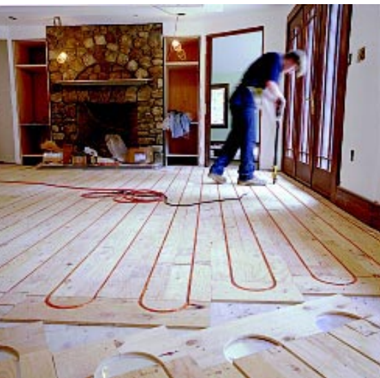
The Stadler method of under-floor heating is ideally suited to the American tradition of building houses from wood.
