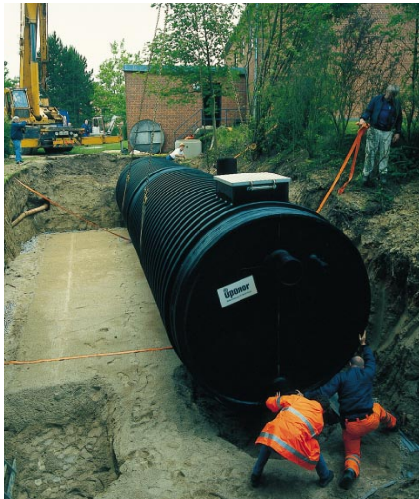
Care of the environment creates a demand for new products. Above is a large Uporol container, which is being installed to collect rain and flood water in Denmark. When the water is collected in this way, it can be released back into the watercourses more slowly and naturally. Local residents also benefit by being able to use the collected water free of charge for watering their vegetable plots.
