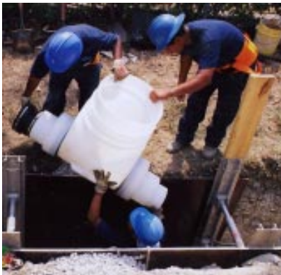
The inspection chamber for sewer pipes is one of the newest products at Uponor ETI. The design has undergone a series of modifications to ensure that it exactly matches end-user requirements.
