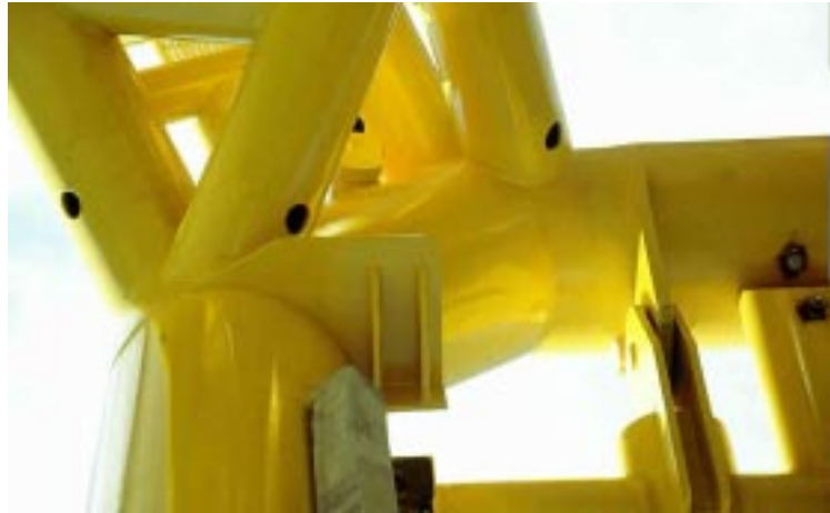
Heavy pipes manufactured by Rautaruukki Steel's Presteel Oy for the undersea protective structures of an oil-drilling platform.
