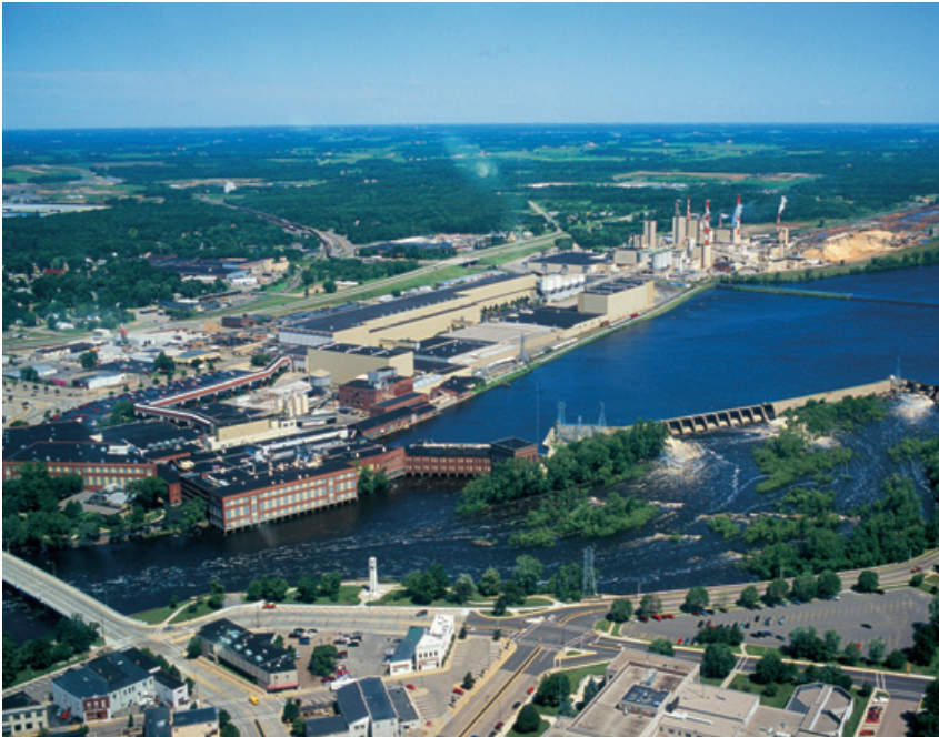
Wisconsin Rapids mill site.
