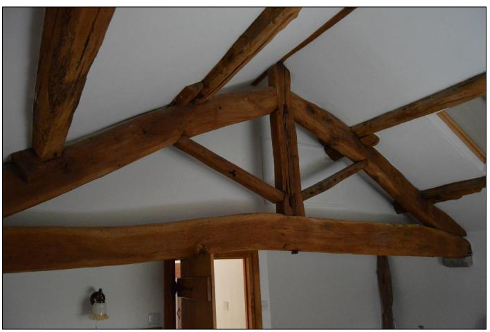
PL17: View of the timber king post roof truss to the first-floor bedroom.
