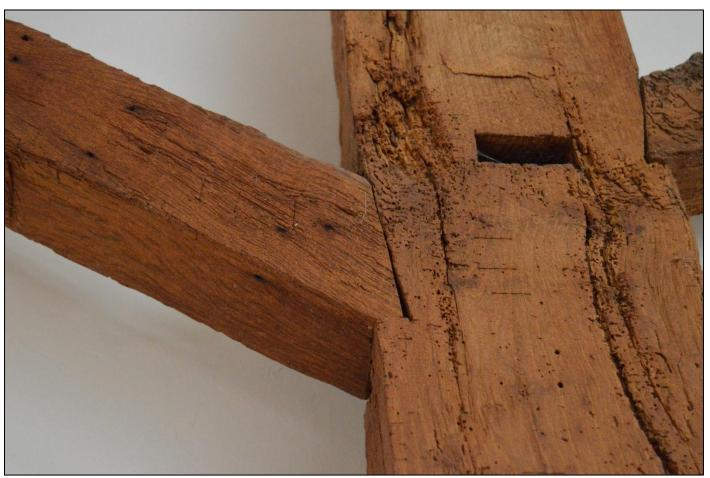
PL21: View of carpenters' assembly marks to the landing truss.
