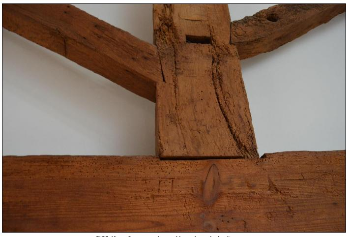
PL22: View of carpenters' assembly marks to the landing truss.
