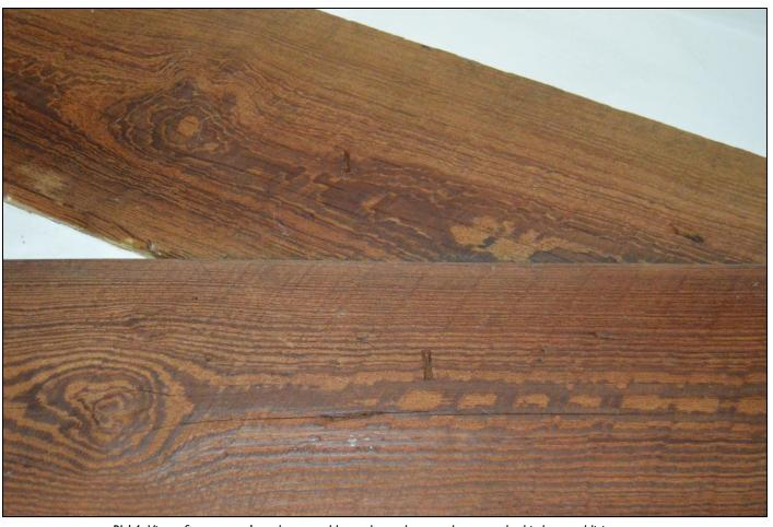
PL14: View of carpenters' marks assembly marks to the truss between the kitchen and living room.
