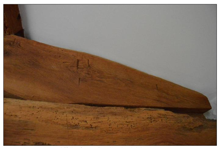
PL23: View of carpenters' assembly marks to the bedroom truss.
