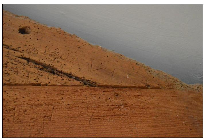
PL19: View of carpenters' assembly marks to the landing truss.
