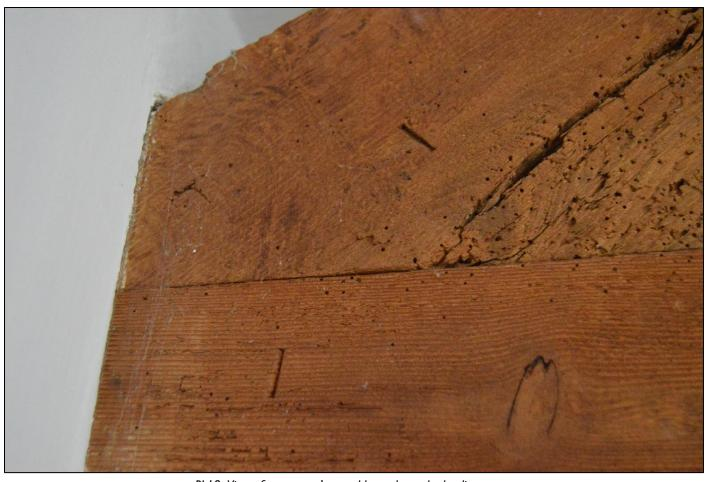
$\label{eq:plished} \textit{PL18: View of carpenters' assembly marks to the landing truss.}$
