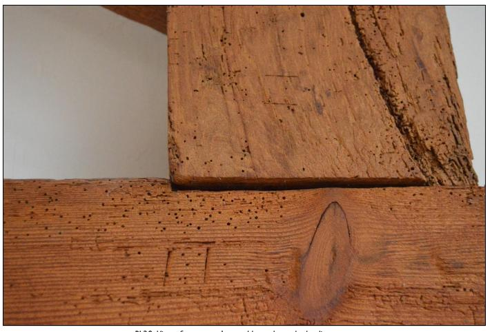
PL20: View of carpenters' assembly marks to the landing truss.
