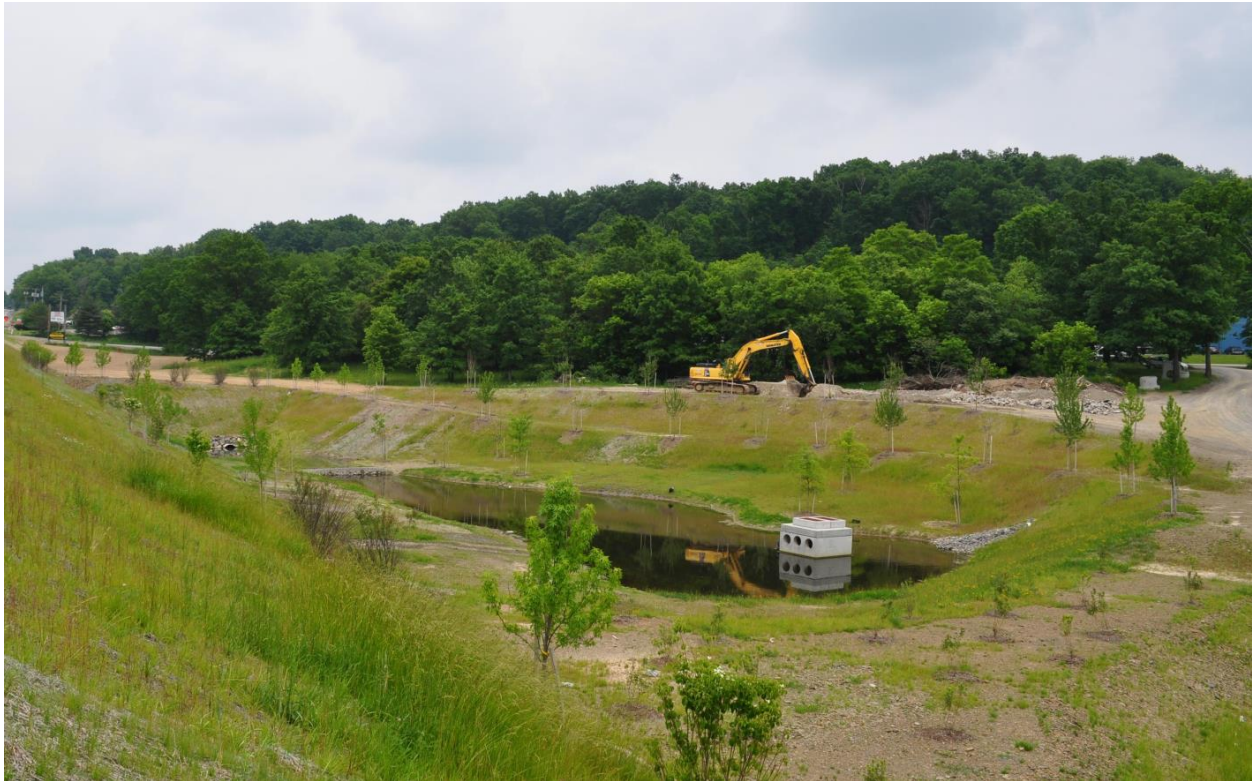
Figure 6.2.1: Newly Constructed Wet Detention Basin (photo c/o: PennDOT)
