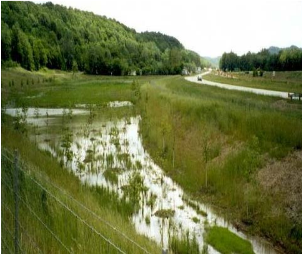
Figure 6.7.1: Stormwater Wetland – Extended Detention Shallow Wetland (photo c/o: PennDOT)
