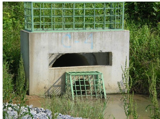
Rectangular weir & circular orifice with trash rack
