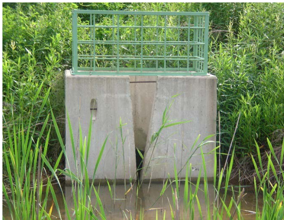
V-notch weir with top mounted trash rack
