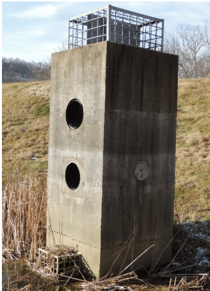
Circular orifices with trash rack on low flow orifice and top
