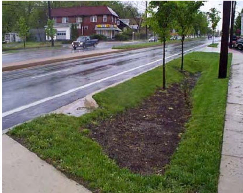
Figure 6.5.1: Subsurface Infiltration Trench (photo c/o: PennDOT)
