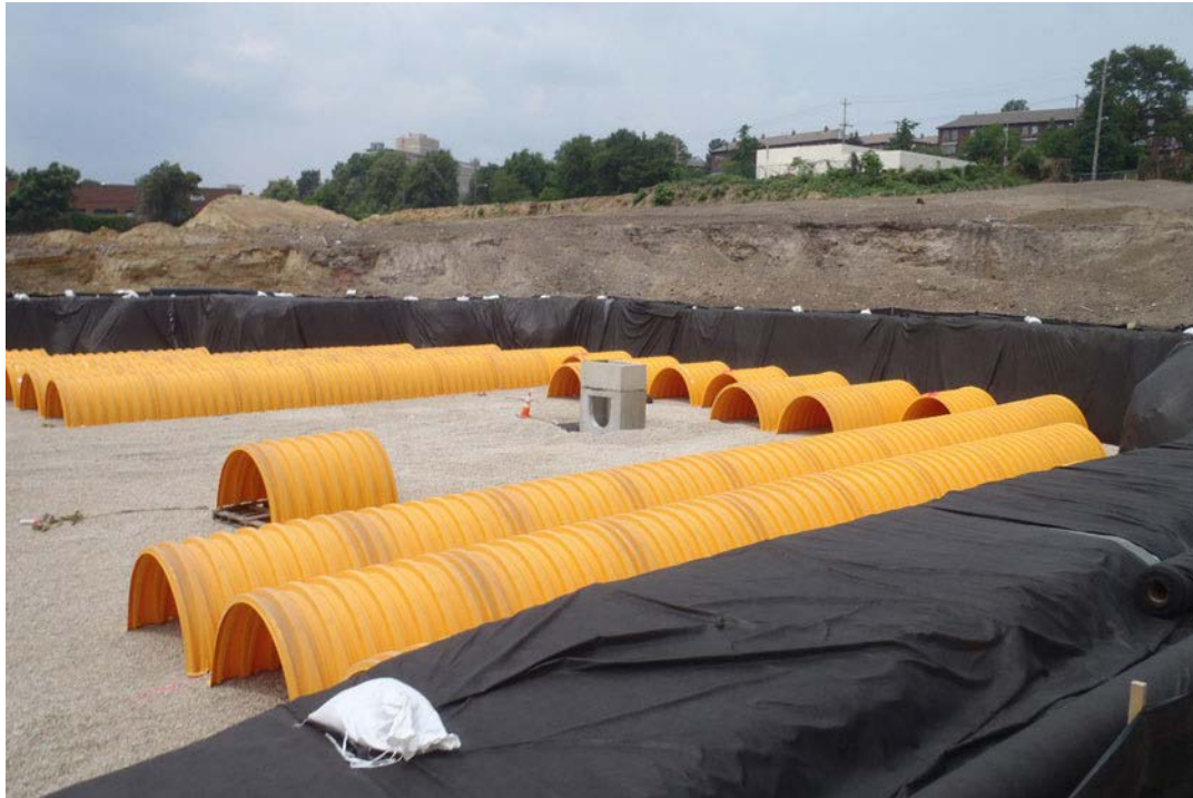
Figure 6.6.1: Subsurface Detention Storage Under Construction
