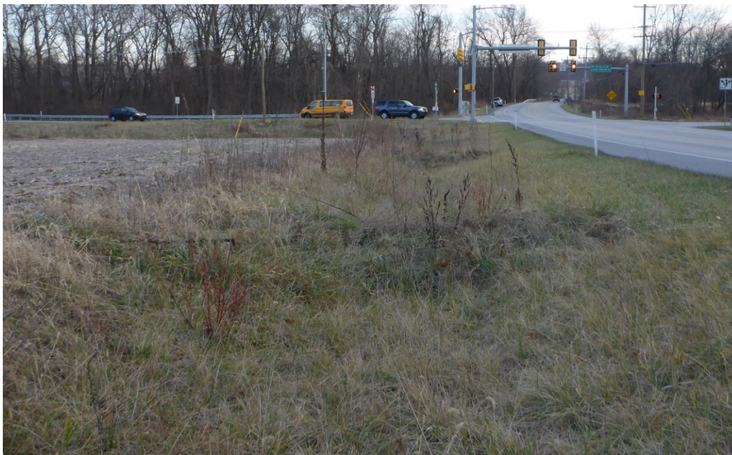
Figure 6.11.2: Vegetated Swale with Check Dams (VSC)
