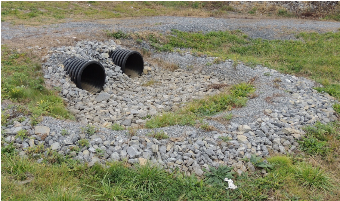
Forebay with Rock Surface
