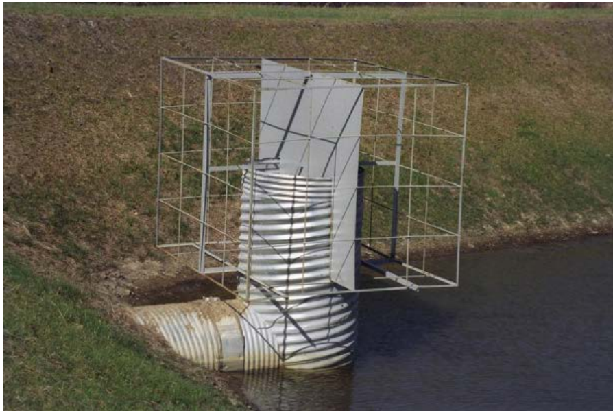
Metal Riser with Trash Rack and Vortex Plate (photo c/o: PADEP E&S Manual)
