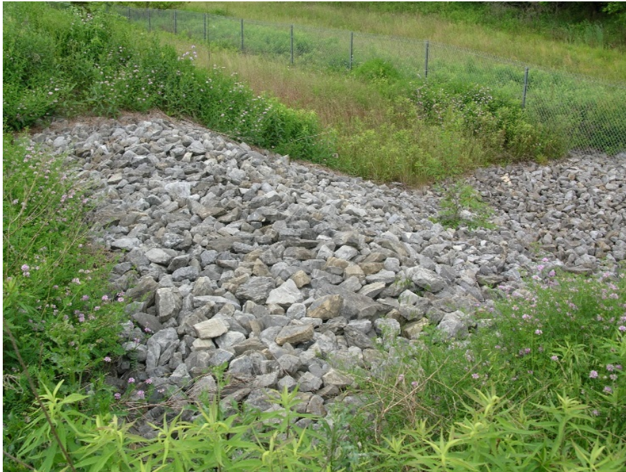
Figure 5.10.1: Emergency Spillway (photo c/o: PennDOT)
