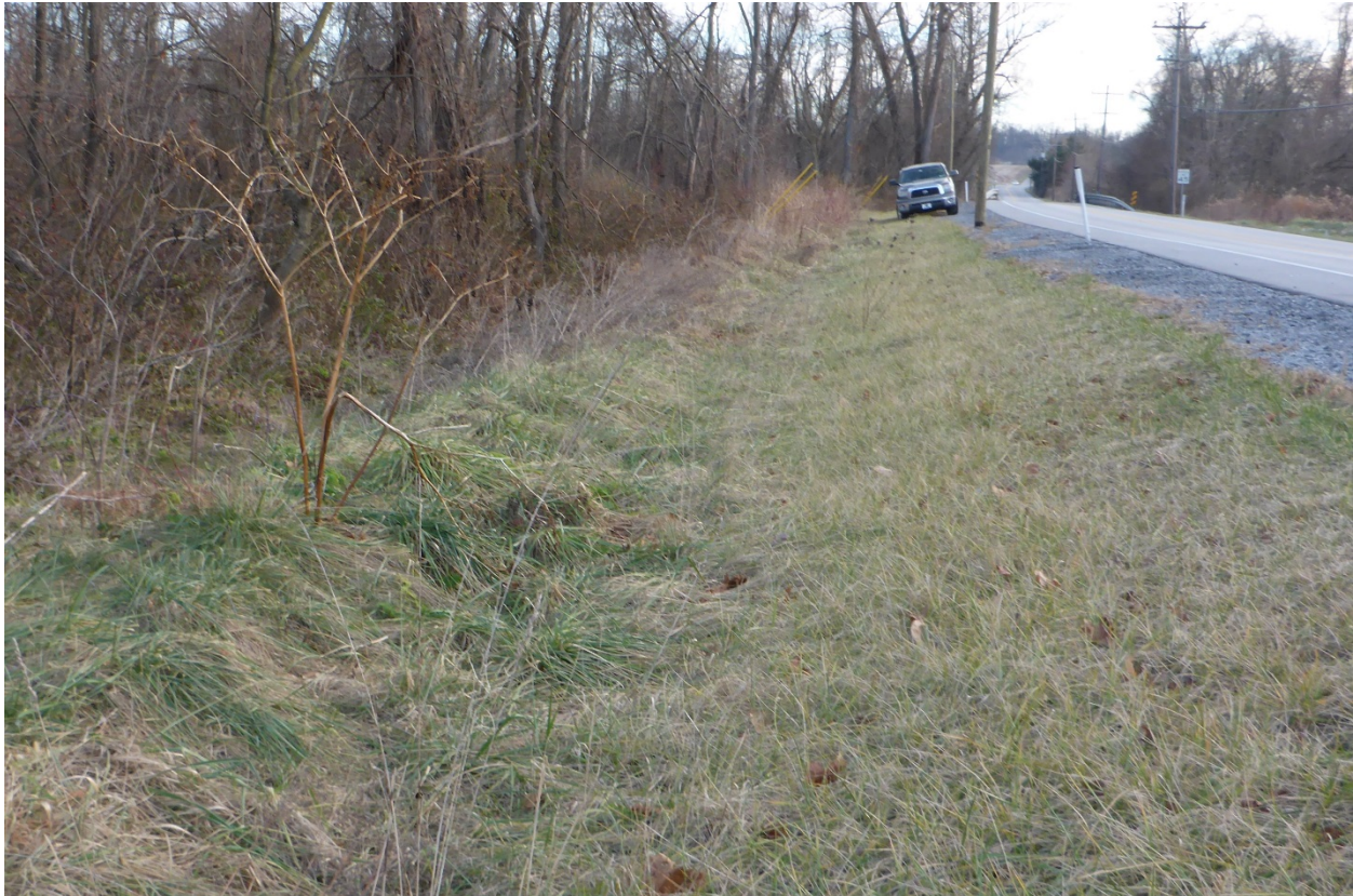
Figure 6.12.1: Infiltration Berm (photo c/o: PennDOT)
