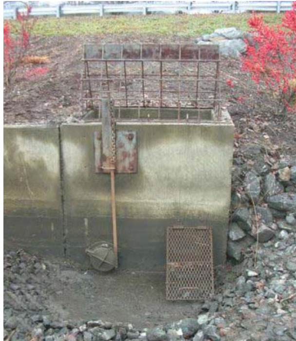
Figure 6.2.3: Lift-Type Sluice Gate (c/o NCDot-HSP-2010-01)
