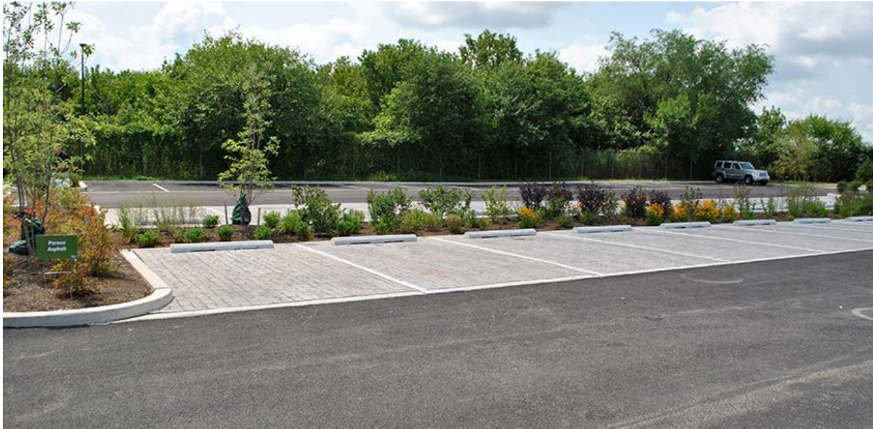
Figure 6.15.1: Pervious Pavement Pavers (PPP)
