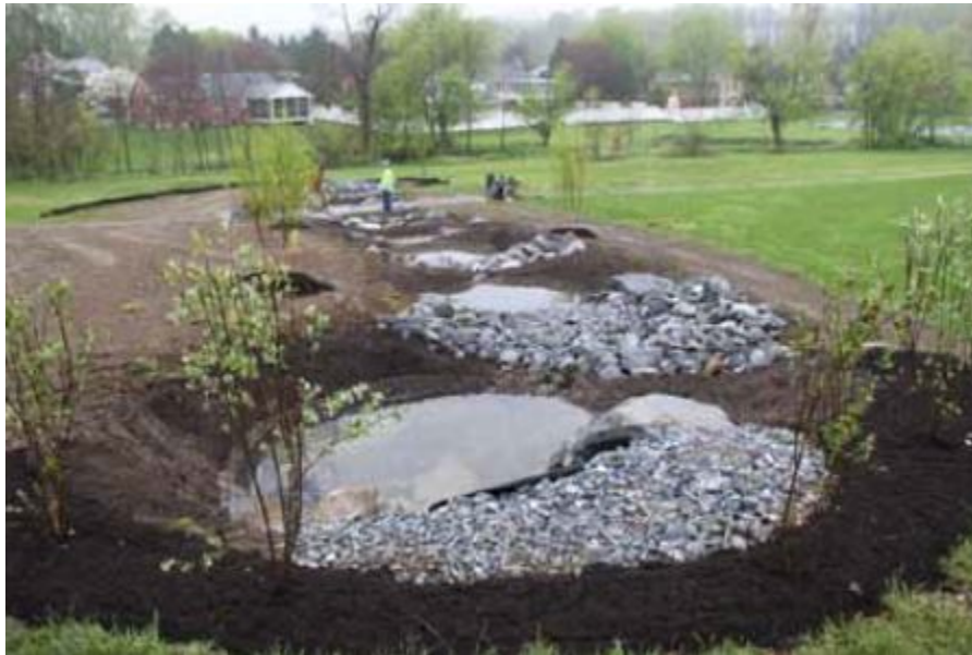
Figure 6.16.1. Regenerative Step Pool (newly constructed; vegetative not fully established) (photo c/o Center for Watershed Protection pilot regenerative step pool project in Lancaster County)
