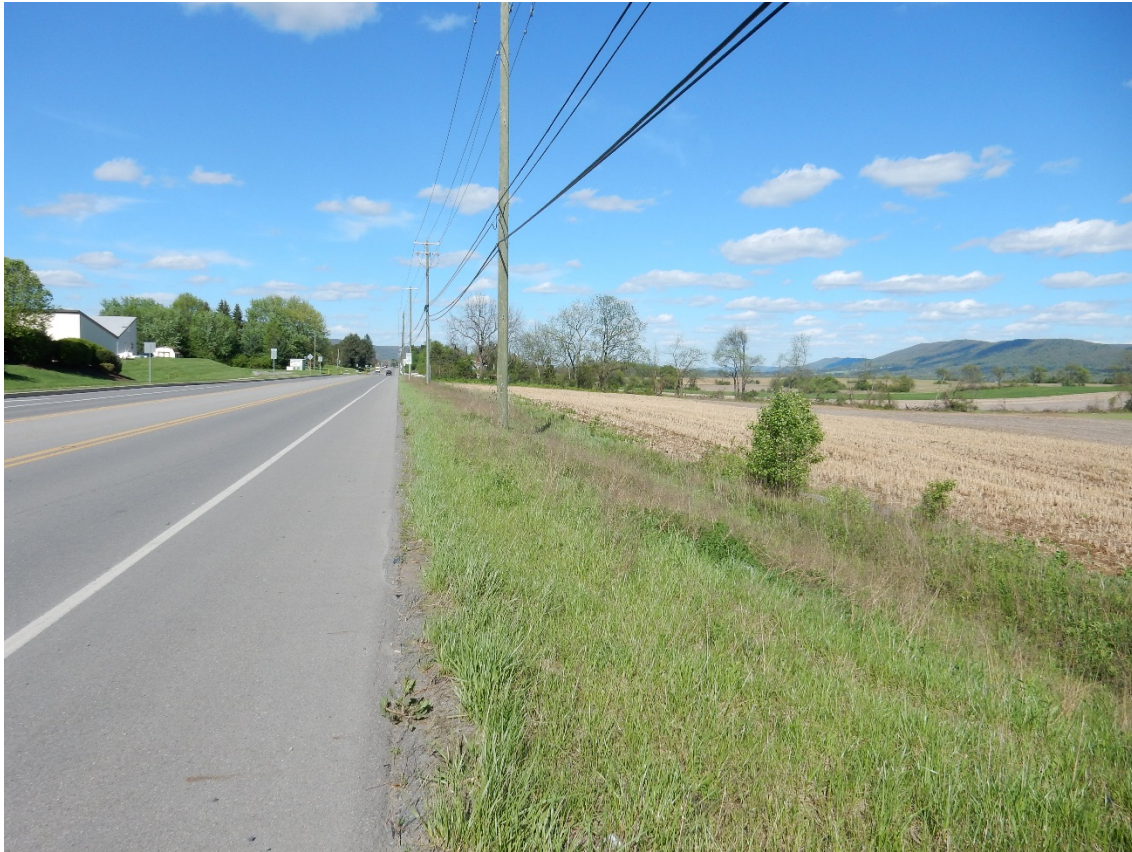
Figure 6.9.1: Vegetated Filter Strip (VFS)
