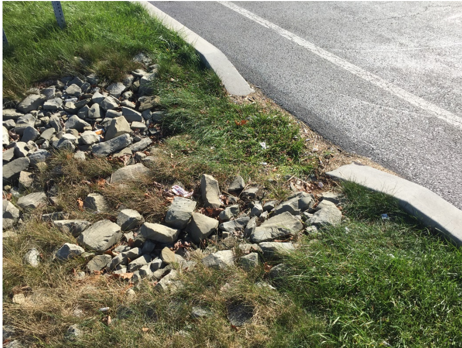
Figure 5.4.1: Inflow System- Curb Cut (photo c/o: PTC)
