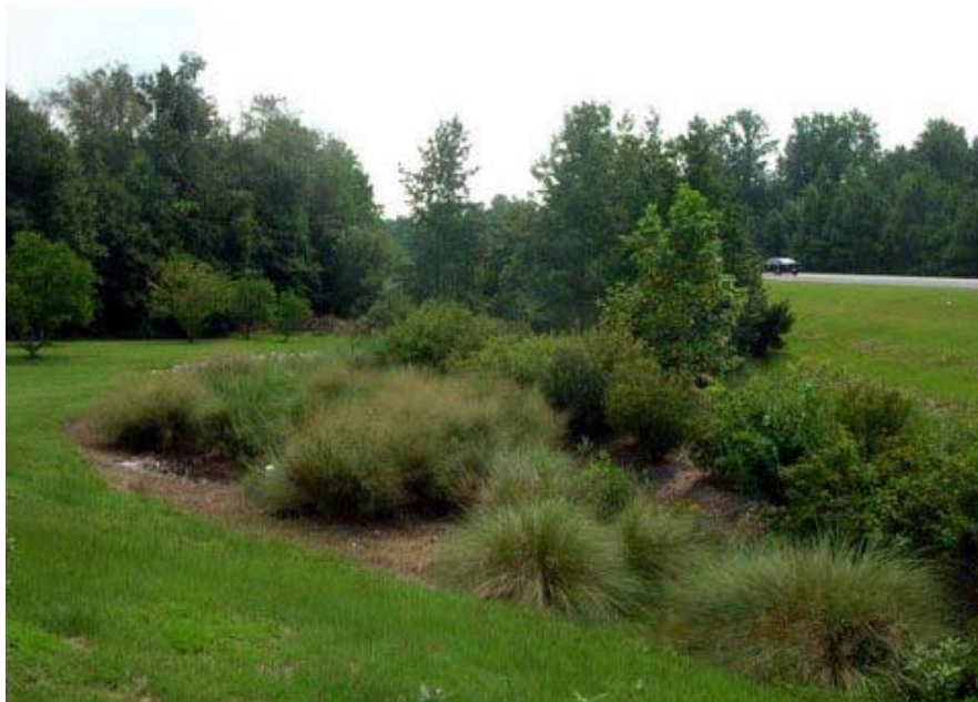
Figure 6.4.1: Bioretention
