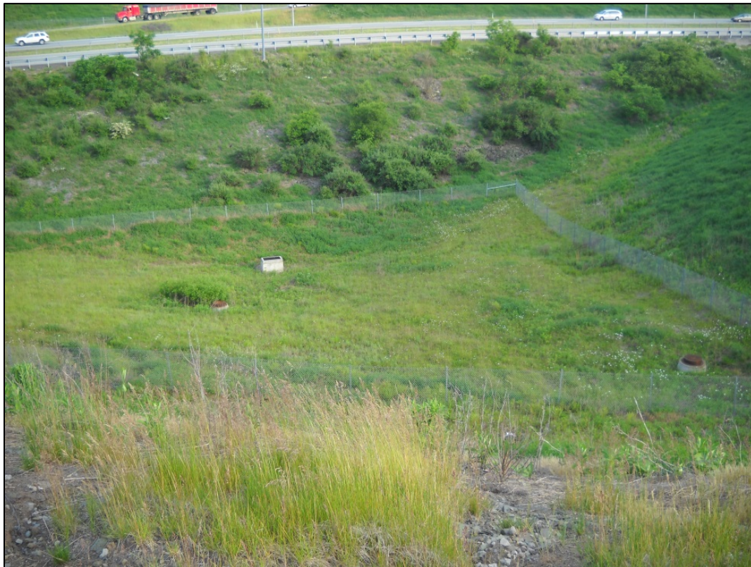
Figure 6.1.1: Dry Extended Detention Basin (photo c/o: PennDOT)
