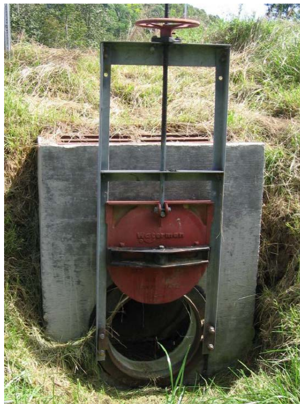
Figure 6.2.4: Open Screw-Type Sluice Gate (c/o NCDot-HSP-2010-01)
