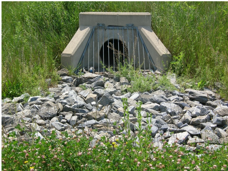
Endwall with Trash Rack (photo c/o: PennDOT)
