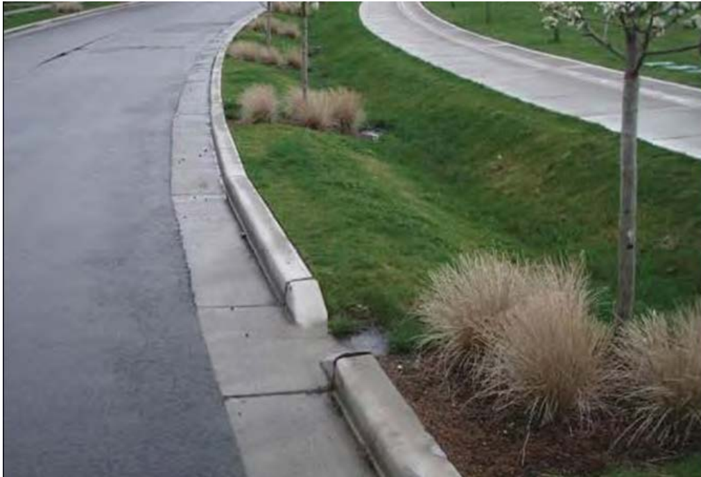
Figure 6.11.1: Vegetated Swale (VSW)
