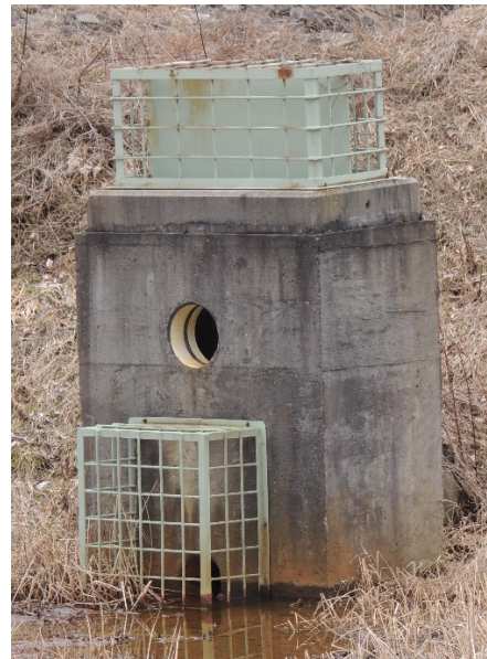
Circular orifices with trash rack on low flow orifice and top
