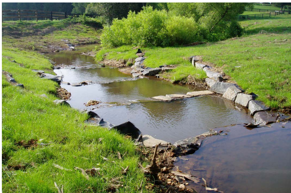
Stream Restoration- Cross Vane Structures
