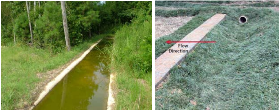
Figure 6.14.1: Level Spreader, Surface Type (photo on left c/o NCDOT HSP-2010-01; photo of right c/o NCSU)
