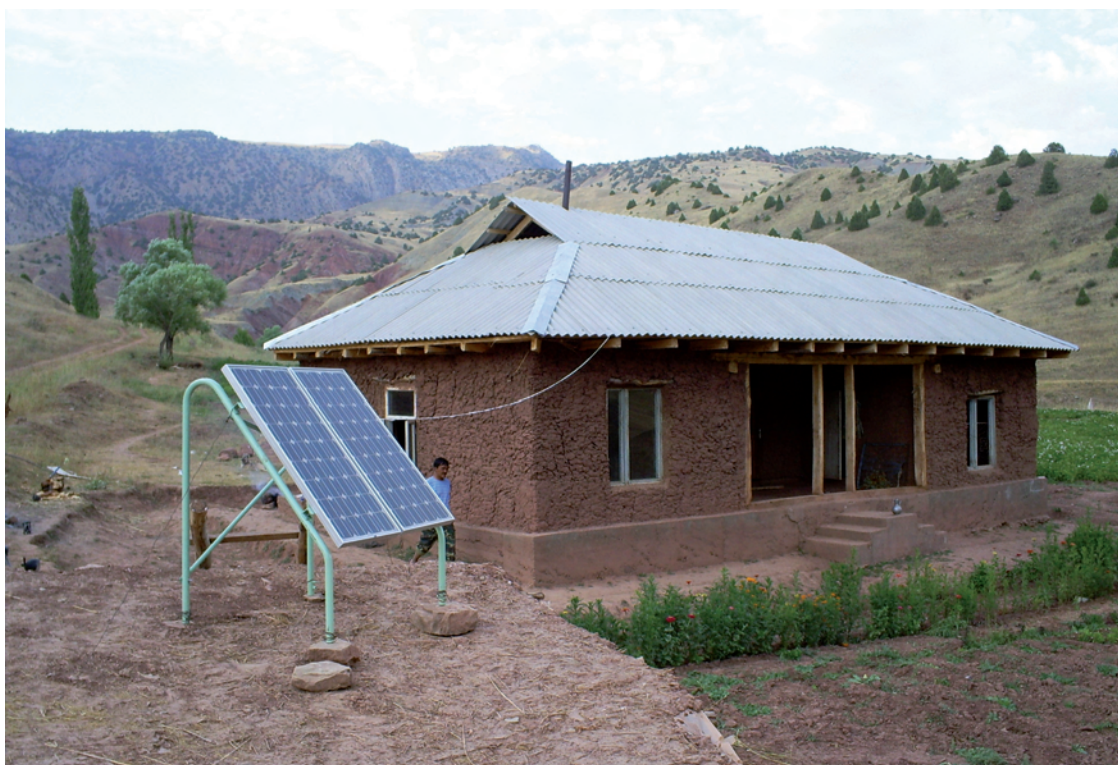
Kashkadarya region. Domestic photoelectric station in Gissar reserve
