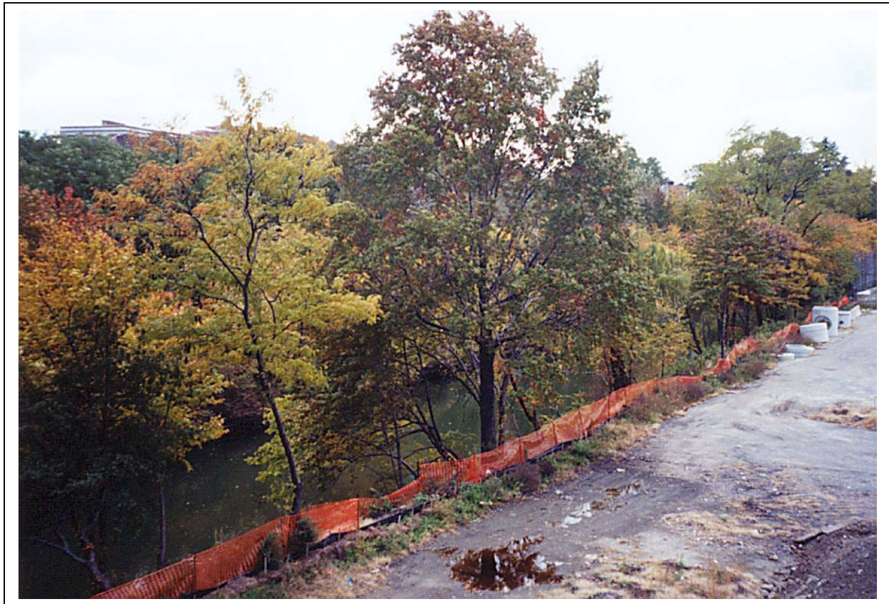
Figure 3.4 Restoration efforts underway near the Bronx River at 174 th Street.
