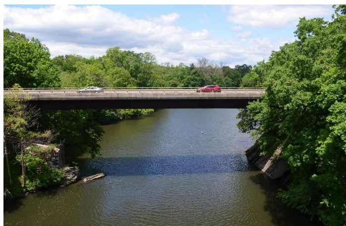
Figure 33: Still River Road, New Milford Bridge Crossing Housatonic River
