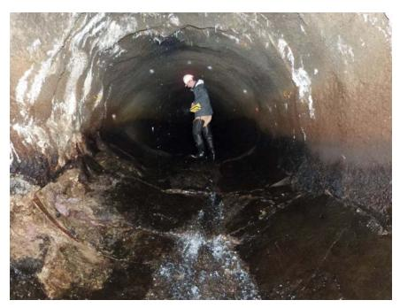
**FIGURE 2.11** Photo of heave in the tunnel. The tunnel diameter was originally 11 feet. The man is standing on the heaved portion of the tunnel. SOURCE: Britton et al., 2016a.
