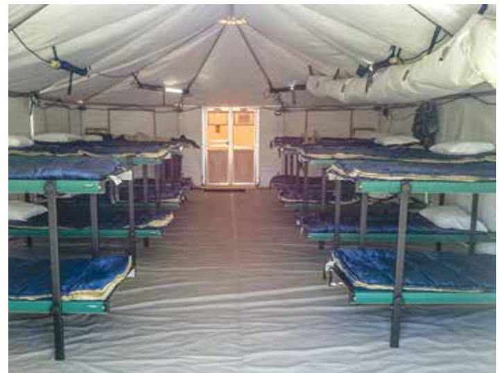
Shelter billeting featuring Western Shelter bunk beds, air distribution plenum, lighting and wiring harness.
