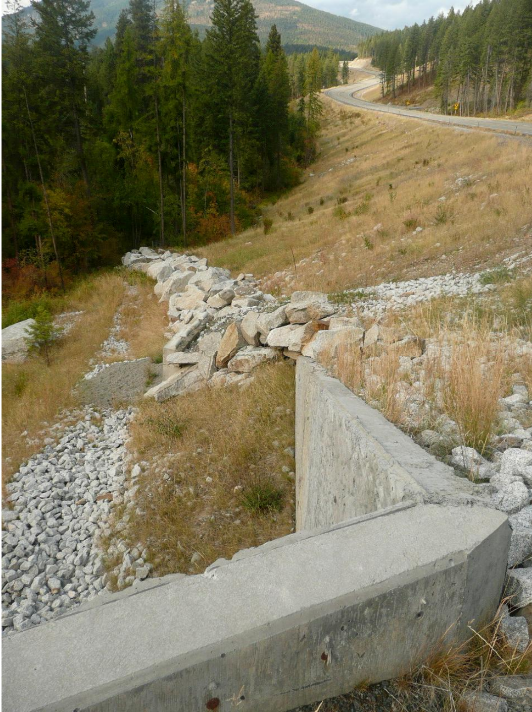
Exhibit 7. Wing wall at wildlife underpass and connection to large boulders, substituted for wildlife exclusion fence on west-side of US 95, near Bonners Ferry, Idaho. (copyright: Tony Clevenger)
