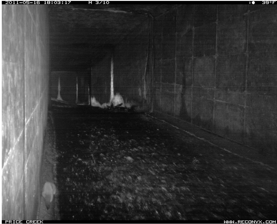
A mink venturing into the Price Creek Culvert during high water flow. The mink, the first detected in this culvert, aborted two apparent crossing attempts within a 30-minute period. (Photo: WTI)
