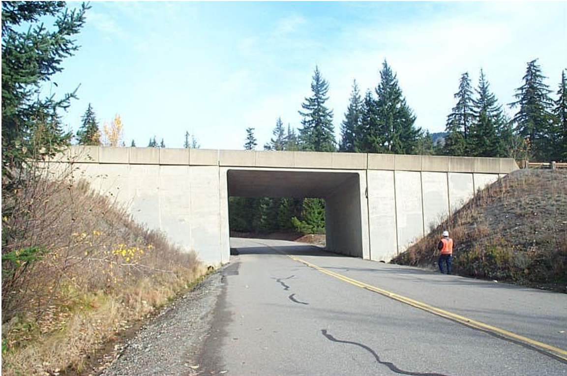
Sparks Road Bridge South. (Photo: WSDOT)
