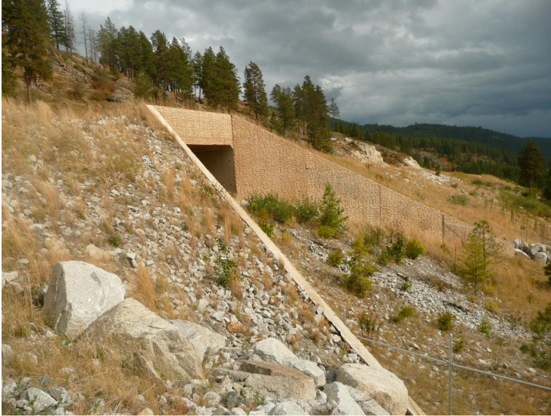
Exhibit 11. Retaining wall at wildlife underpass on US 95 near Bonners Ferry, Idaho. (copyright: Tony Clevenger).
