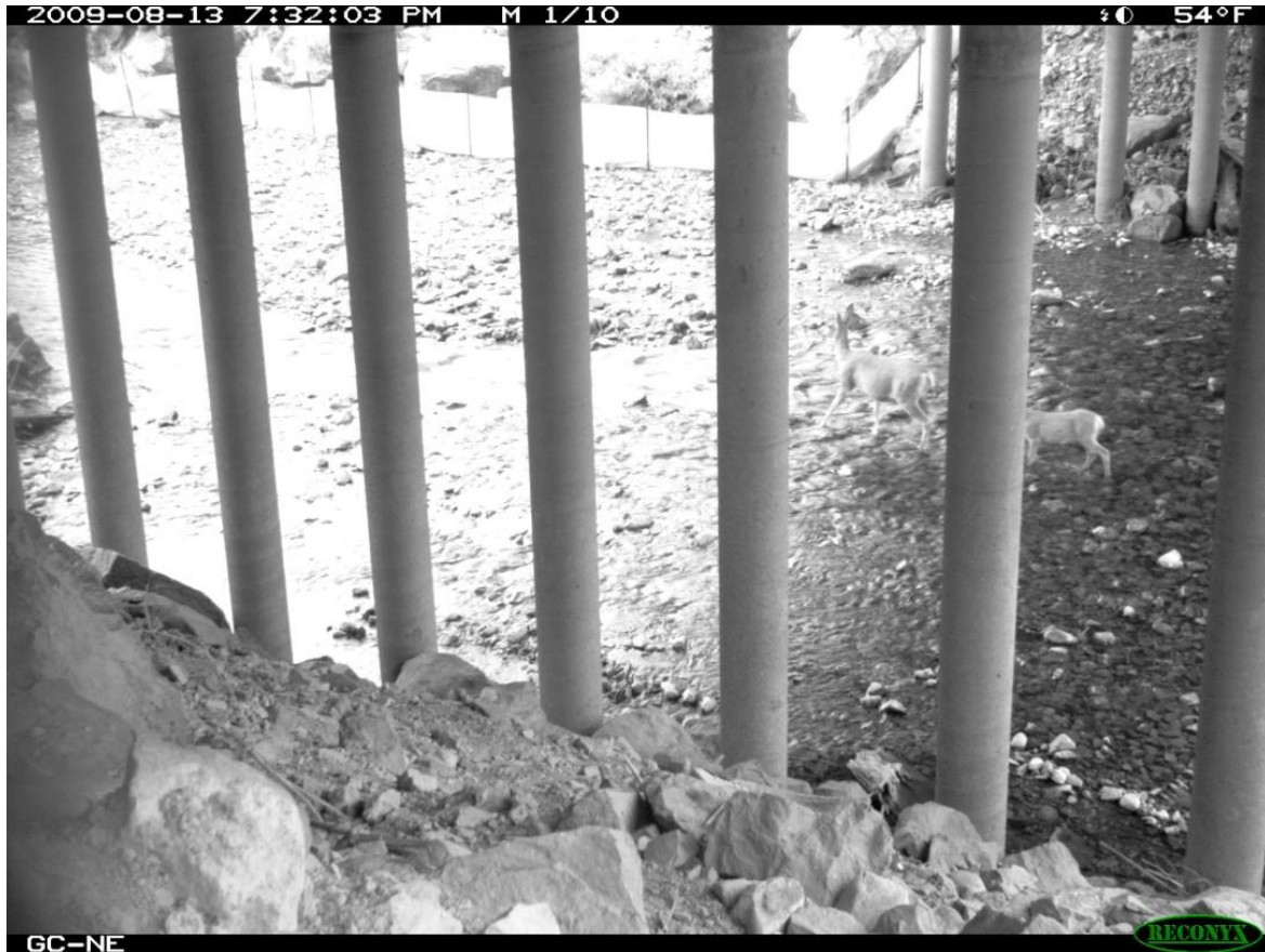
An adult deer and fawn pass from north to south under the Gold Creek North Bridge. (Photo: WTI)
