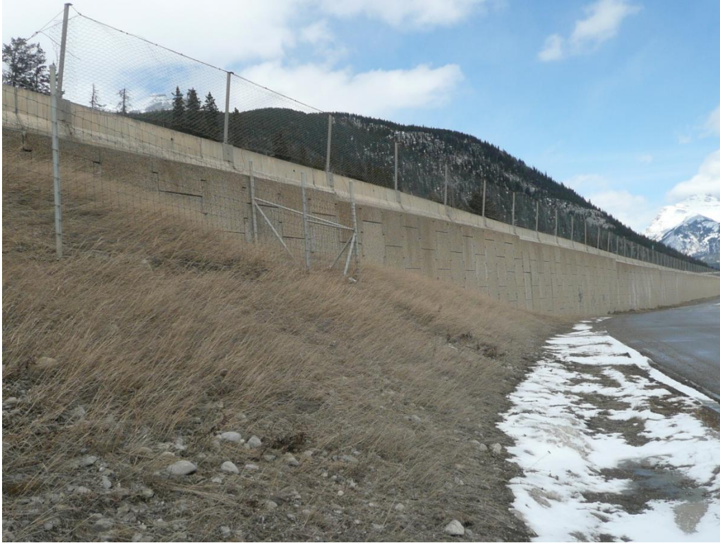
Exhibit 5. Mechanically stabilized earth (MSE) retaining wall along the Trans-Canada Highway in Banff National Park, Alberta. (copyright: Tony Clevenger)
