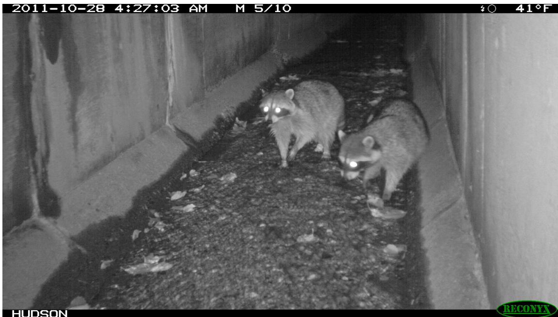
HUDSON Raccoons cross through Hudson Creek Culvert. (Photo: WTI)
