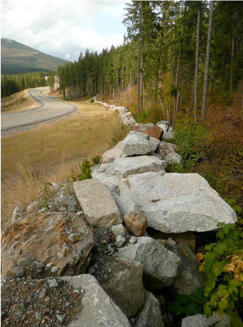
Exhibit 6. Boulder wall substituted for wildlife exclusion fence on eastside of US 95, near Bonners Ferry, Idaho. (copyright: Tony Clevenger)
