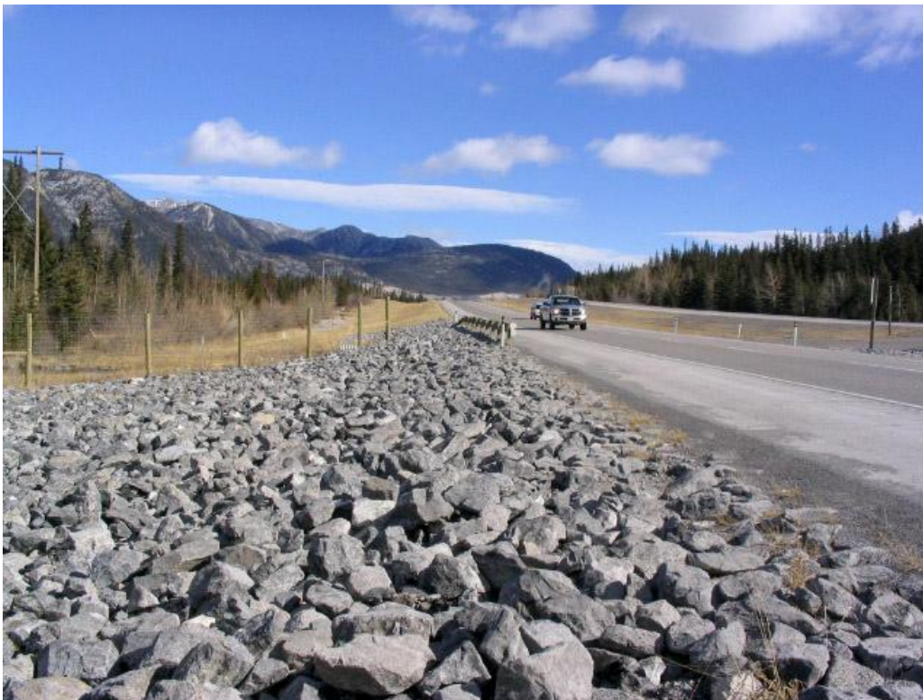
Exhibit 10. Boulder field at termination of wildlife fence on Trans-Canada Highway, near Canmore, Alberta (copyright: Tony Clevenger).
