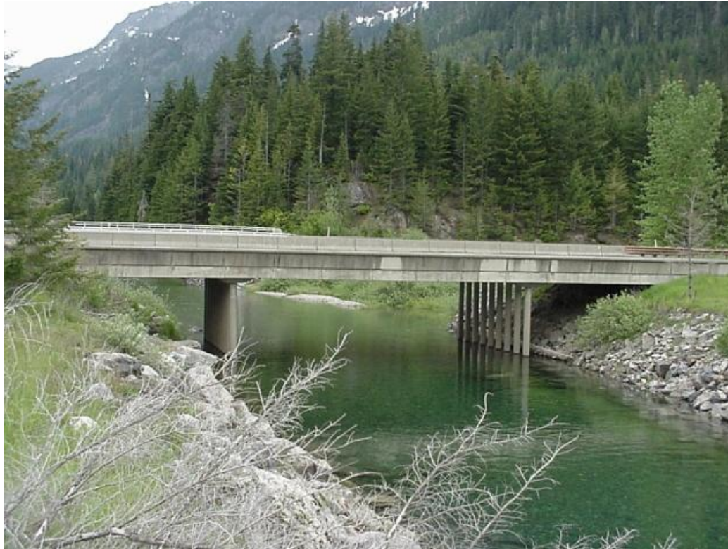
Gold Creek Bridge NE (right bank) and NW (left bank). (Photo: WSDOT)
