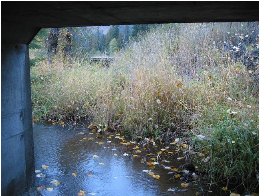
North entrance of Swamp Creek West Culvert. (Photo: WTI)
