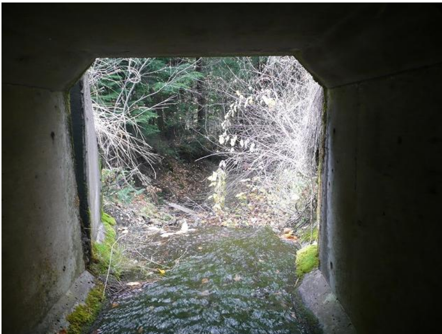
Cedar Creek Culvert north entrance. (Photo: WTI)
