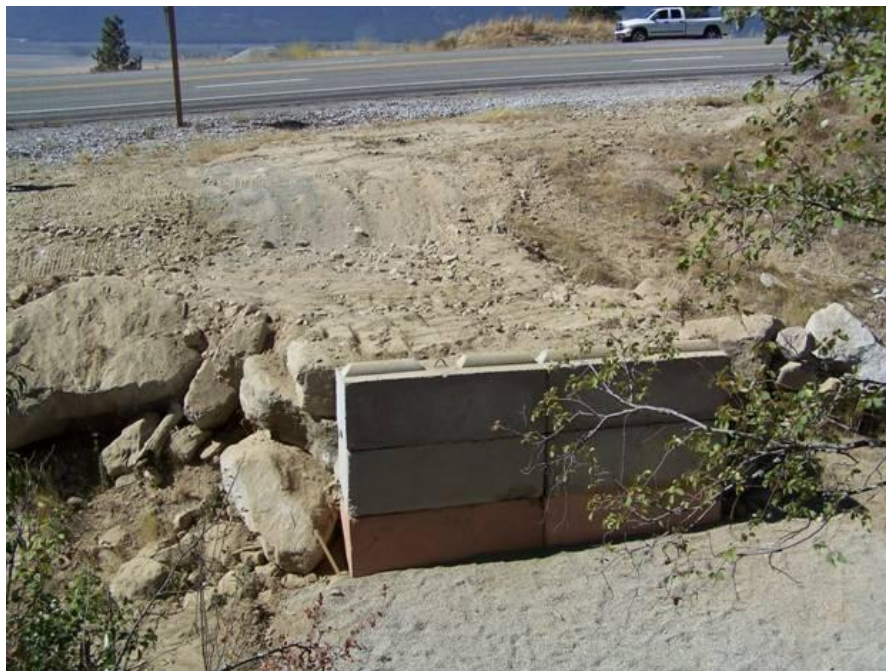
Exhibit 8. Escape ramps on US 95 near Bonners Ferry, Idaho. (a) Lateral view of escape ramp fitted into boulder wall on downhill side of highway; (b) elevated view of escape ramp under construction with landing pad in place. (copyright: Tony Clevenger [a] and Wayne Wakkinen [b])
