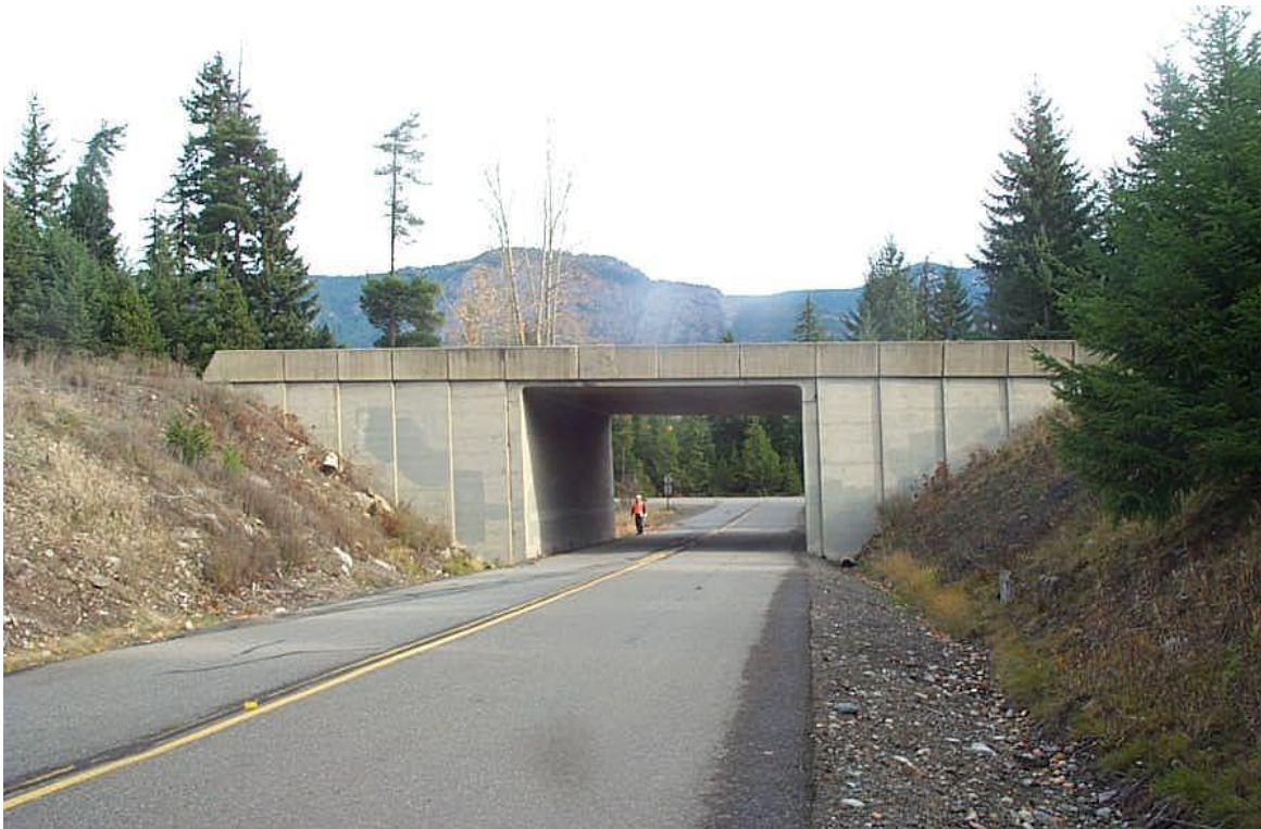
Sparks Road Bridge North. (Photo: WSDOT)
