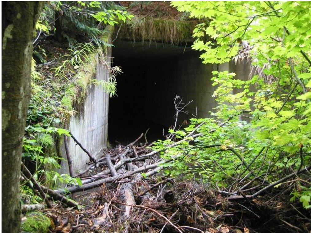
Price Creek Culvert north entrance. (Photo: WTI)
