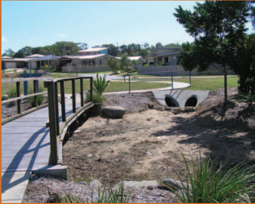
Stormwater run-off control in a Mackay housing estate that is designed to minimise impacts to surrounding coastal and sub-coastal tree swamps Photo: Kylie Joyce, DERM
