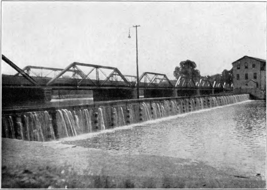
A.—GOVERNMENT DAM ACROSS THE FOX RIVER AT MENASHA Head, about 9 feet; 2400 horsepower developed at ordinary flow.
