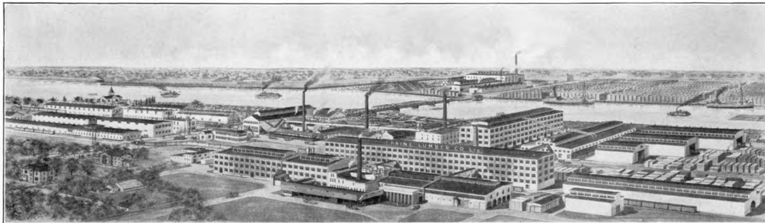
PLANT OF THE PAINE LUMBER COMPANY, OSHKOSH One of the largest manufacturing establishments in the Fox River Valley.
