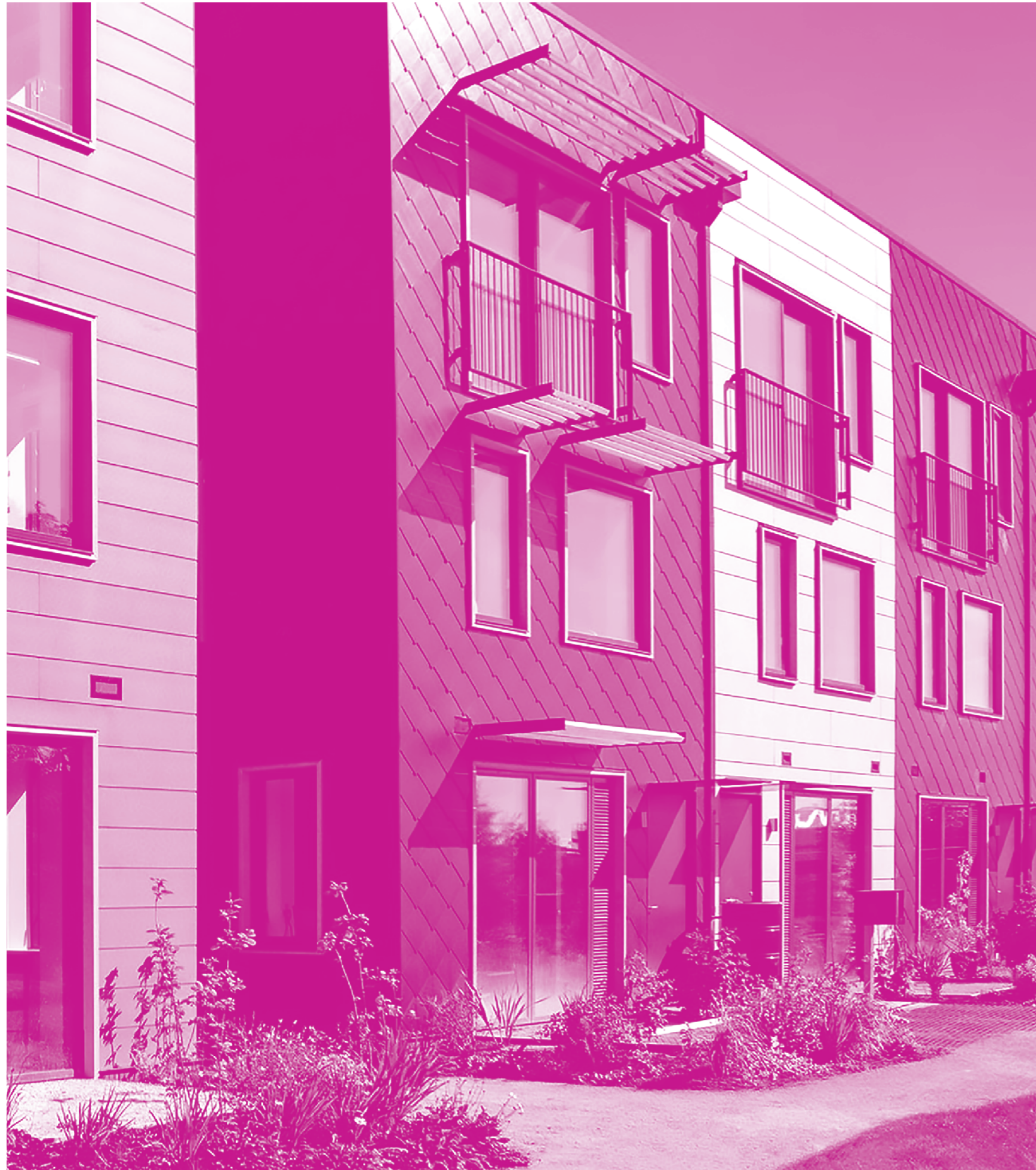
Solar Avenue in the Climate Innovation District in Leeds, consists of 60 town houses with low climate impact, wooden frame, passive house standard and solar cells. Winner of the Housing Design Award 2020.
