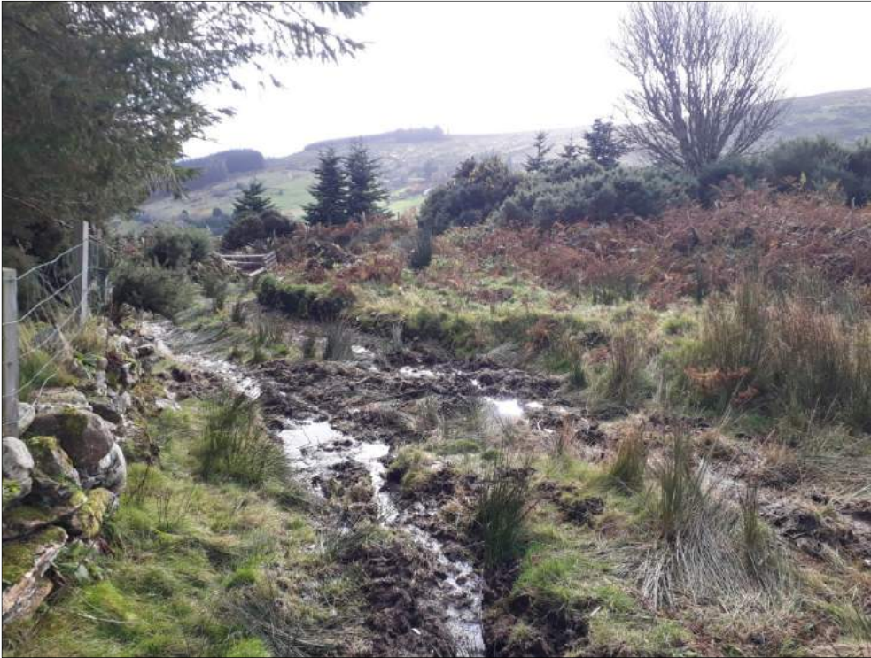
Plate 9. Works to the access lane – will require further work to prevent erosion.
