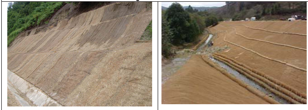
Plate 7.3: Visuals of Use/Installation of Coir-mat to Restore moderate to steep slopes especially along the Road Sides
