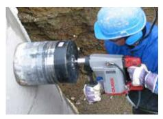
Wet drilling in a concrete shaft, hand-held
