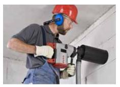
Dry drilling in masonry with dust extraction, hand-held
