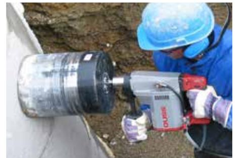
Wet drilling in a concrete shaft, hand-held
