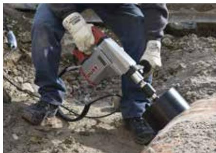
Dry drilling in a plastic pipe, hand-held
