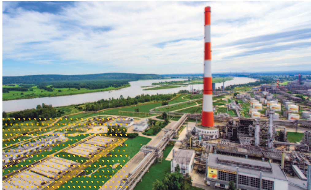
Angarsk Petrochemical Company is building an advanced wastewater treatment facility.
