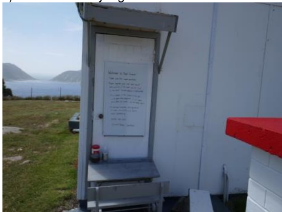
e) Visitor check-in station
