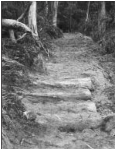
Benching & steps on the new track. Vic. Valley working bee 24/25 April 1999.
