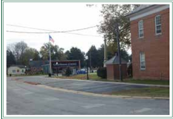
2.28 Old Courthouse Parking
