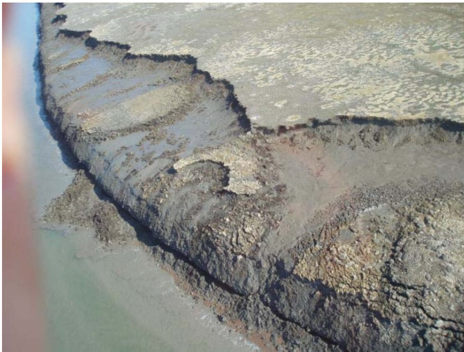
Figure 12. The erosion of the active layer appears to be a result of wave undercuts, infiltration of salt water then mass failure of ice-rich permafrost (photos by S. Carrière 2011).
