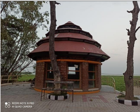
Guard Post ,Jetty ,Car Parking at L.M.B
