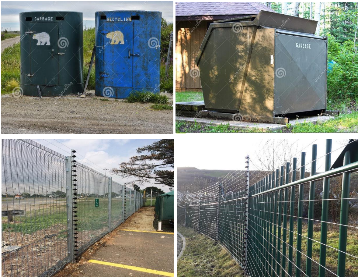
Fig. 33 Shows bear proof garbage bins & perimeter fence
