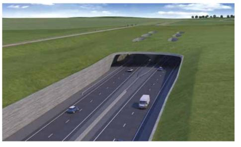
Figure 5.33: Grassed over canopy with ventilation outlets
