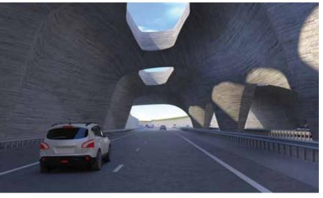
Figure 5.35: Driver's view of canopy with ventilation outlets - exiting
