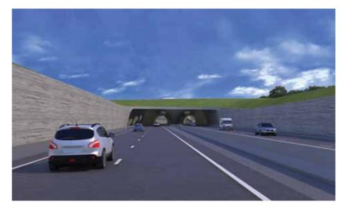
Figure 5.34: Driver's view of canopy with ventilation outlets - entering
