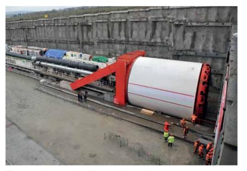
Figure 5.36: An example of the type of tunnel boring machine that would be used
