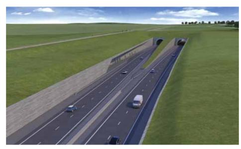
Figure 5.26: Western tunnel entrance - vertical retaining walls option
