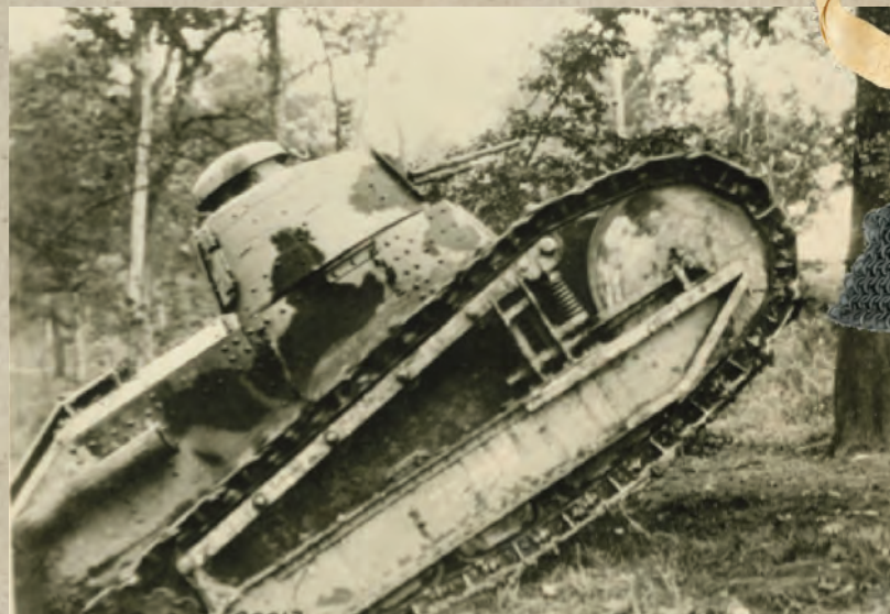
When the U.S. entered the war, it had produced less than one hundred tanks. Borrowing from their French allies, U.S. troops used the newly designed Renault FT light tank for its speed and maneuverability. (WWM Mss 710)
