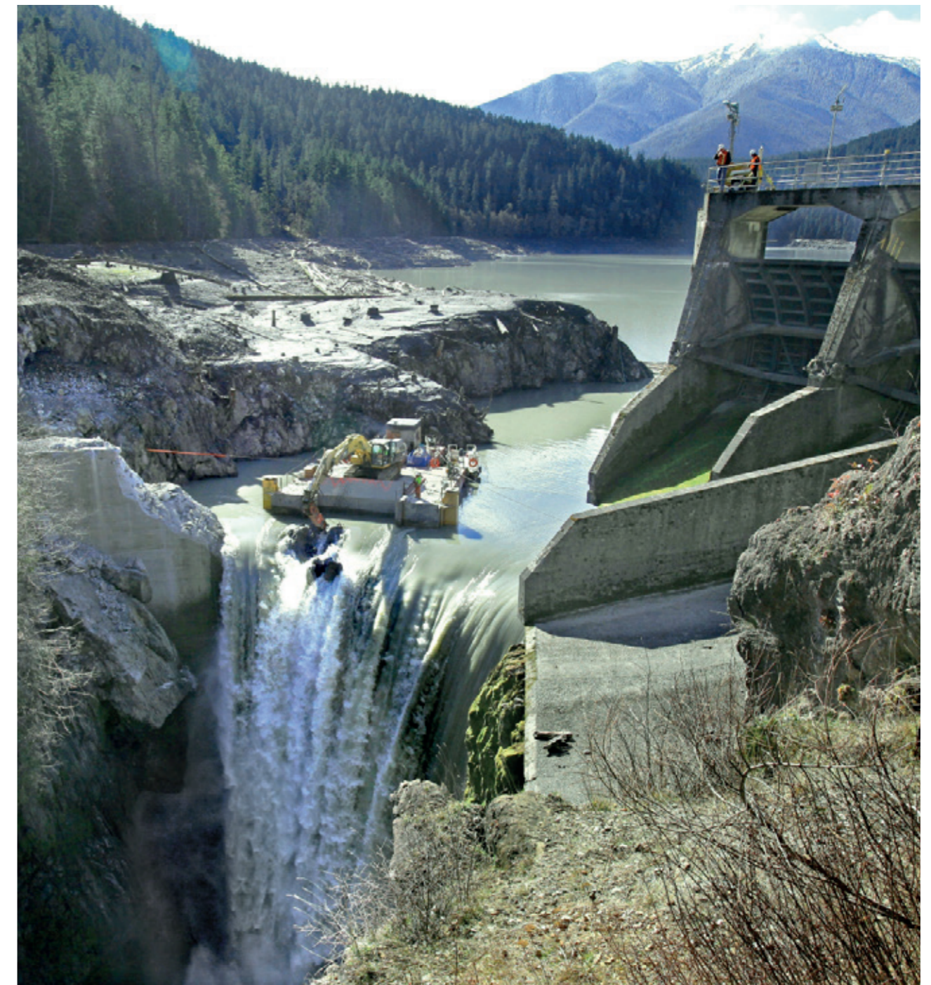
THE 64 M HIGH GLINES CANYON DAM (AKA UPPER ELWHA DAM) DURING REMOVAL
