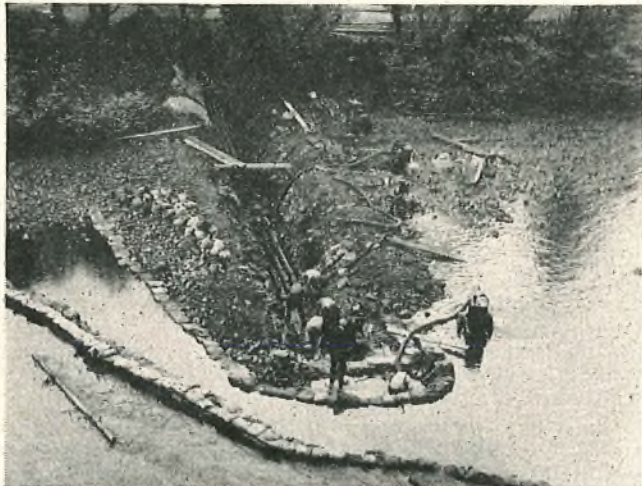
LAYING CAST-IRON PIPES ACROSS THE RIVER TAFF
