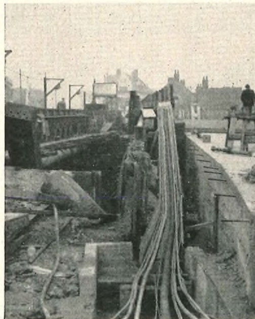
RECONSTRUCTION OF MILL BRIDGE, DONCASTER
