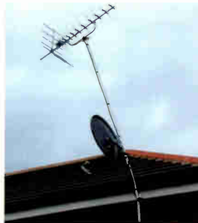
Photo 1 (left): Bill Wright's scrapheap, showing a surprisingly large amount of shiny new metal. Photo 2 (centre): Installed last April, this mast had suffered a trying winter. Photo 3 (right): Installed just seven months ago, this was an accident waiting to happen. A pathetic attempt had been made to support the dish with guy ropes. Note that the DAB aerial is incorrectly polarised, and that the three aerials are much too close together.
