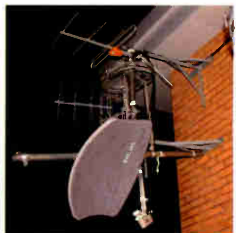
Photo 1 (left): Bill Wright's scrapheap, showing a surprisingly large amount of shiny new metal. Photo 2 (centre): Installed last April, this mast had suffered a trying winter. Photo 3 (right): Installed just seven months ago, this was an accident waiting to happen. A pathetic attempt had been made to support the dish with guy ropes. Note that the DAB aerial is incorrectly polarised, and that the three aerials are much too close together.
