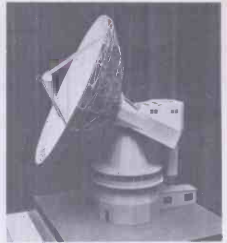
Model of third Goonhilly aerial showing new technique of effectively bringing the ground up to the dish fulcrum.
