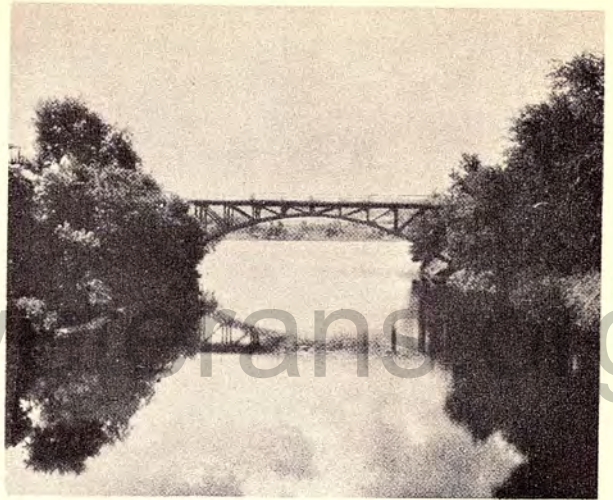
Bridge over Lake Channel on Highway 53.
