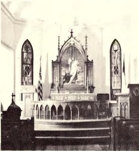
Interior view of Zion Lutheran Church, Galesville
