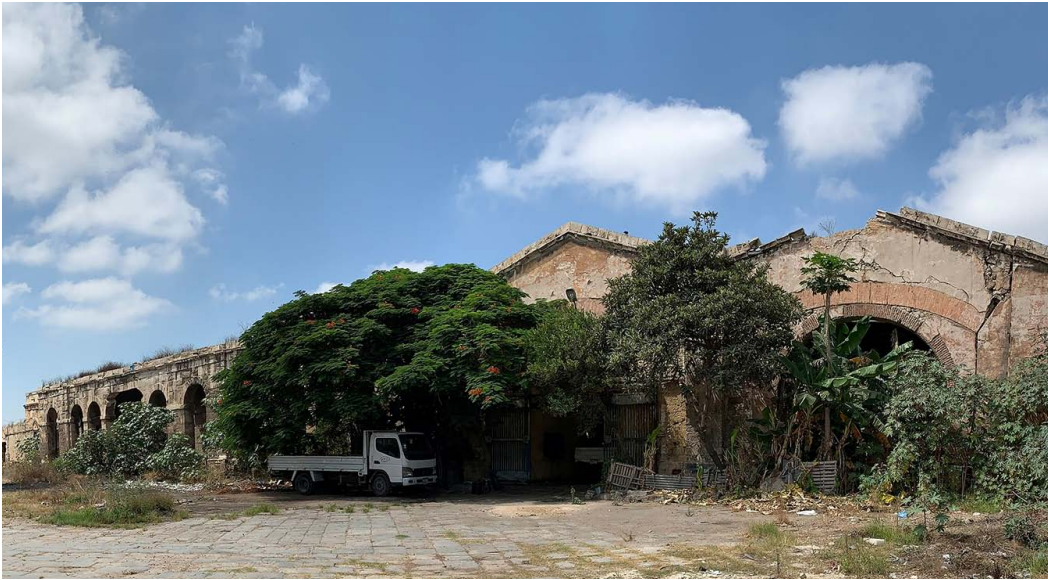
The 1855 Qabbari Railway Station, Alexandria, demolished in early 2022. (Ziad Morsy)
