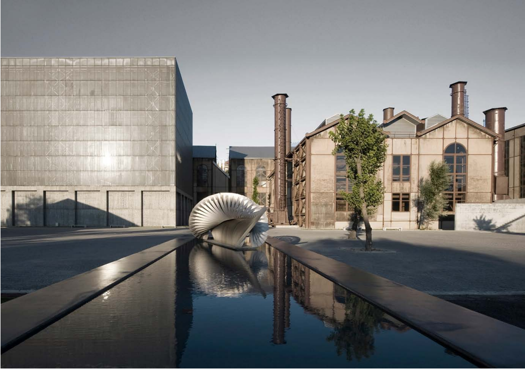
From Silahırađa Power Plant to a center for education, culture and arts of 'santralistanbul' and the main campus of Bilgi University.
