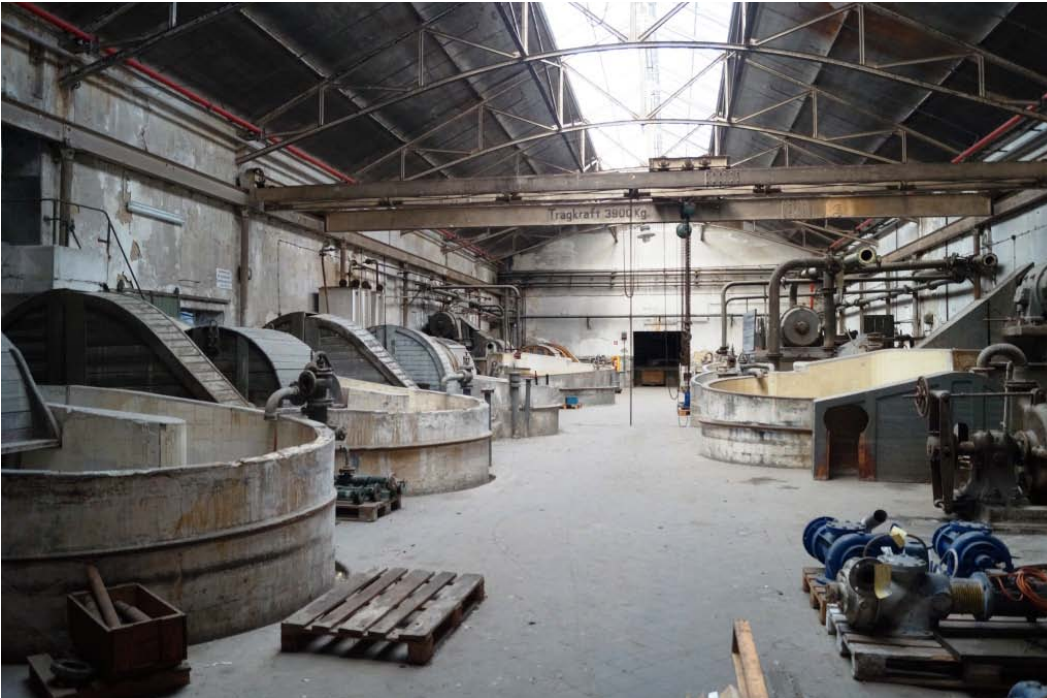
The former Zanders paper mill at Bergisch Gladbach still contains much late-19th century equipment. (Ulrich Schildberg, 2018)
