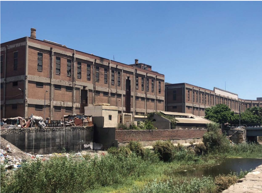
The project to rehabilitate the cotton district and its surroundings in Alexandria (Mirhan Damir)
