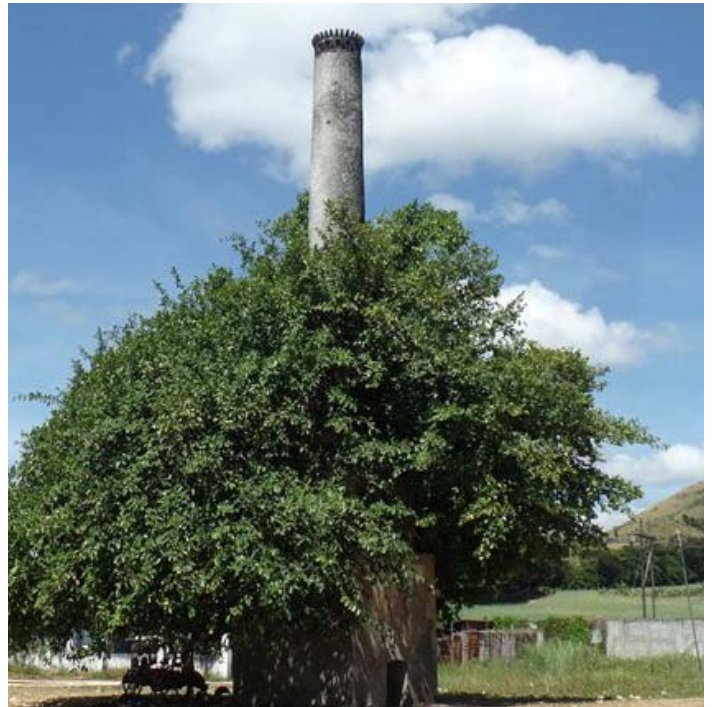
Smokestack of the Ma-ao Sugar Central in Bago City, Negros Occidental and the Sugar Simborios.
