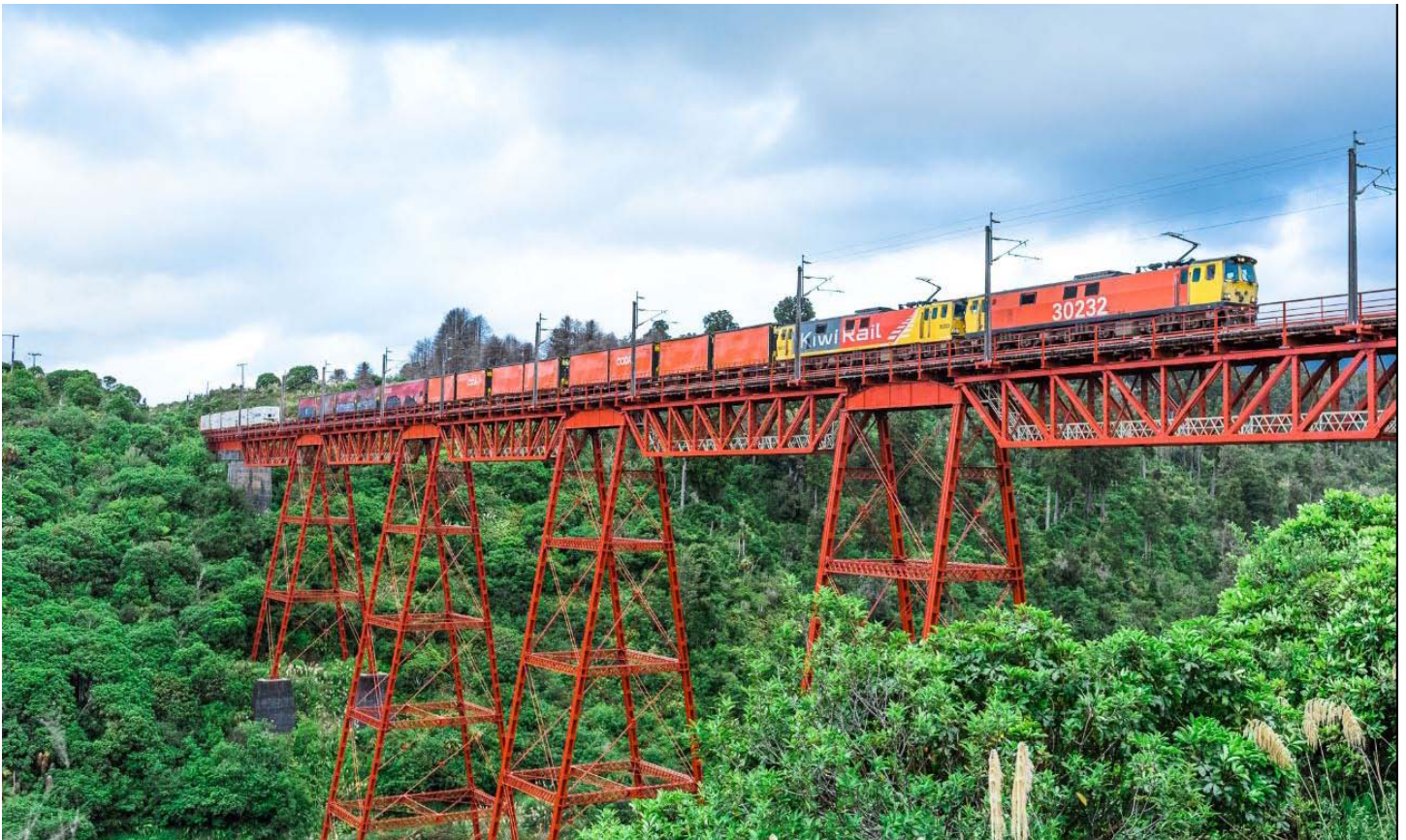
Makatote railway viaduct is recently restored by operator:
