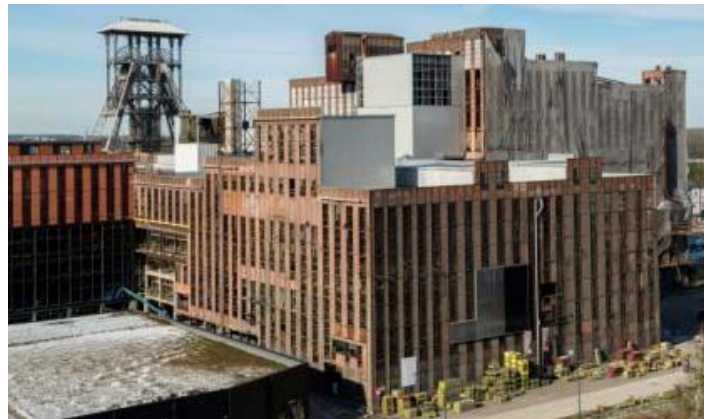
The coal-washing plant of Beringen (Flanders) is the subject of a 'renaturing' proposal. (Bart Vanacker)
