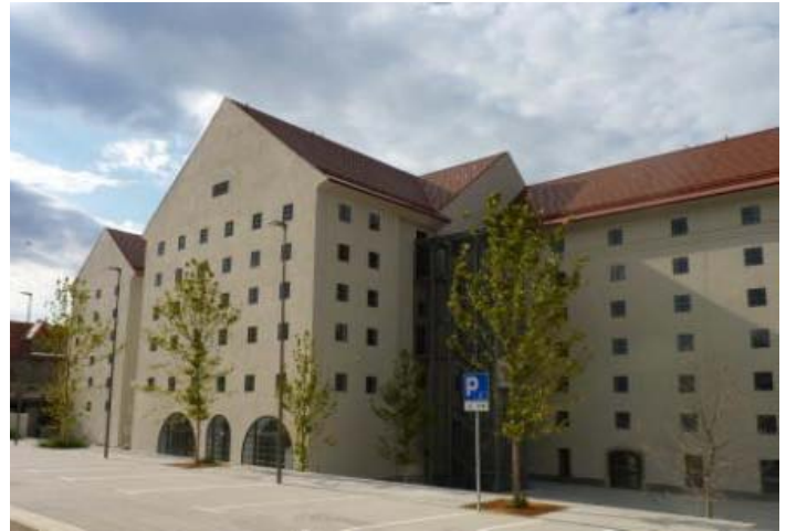
The exterior of the former Cukrarna sugar refinery, now adapted to a cultural centre. (Irena Marušič)
