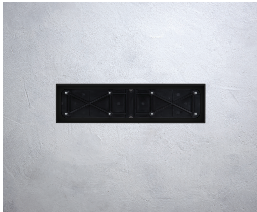
In the example, a cast-in-concrete installation blockout was chosen for site preparation.
