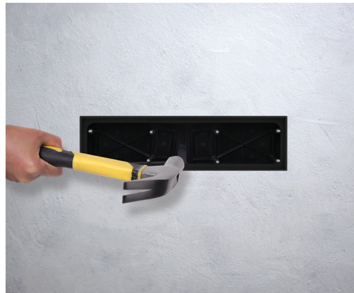
After completion of civil construction, remove the mounting plate in order to access the blockout and mains supply cable(s).
