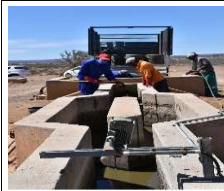
Tanker discharge gives rise to unpleasant odours
