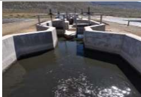
Stuctures are in good condition
