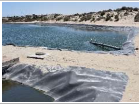
Nine ponds of which 3 are newly constructed. Sections of lining removed by illegal persons
