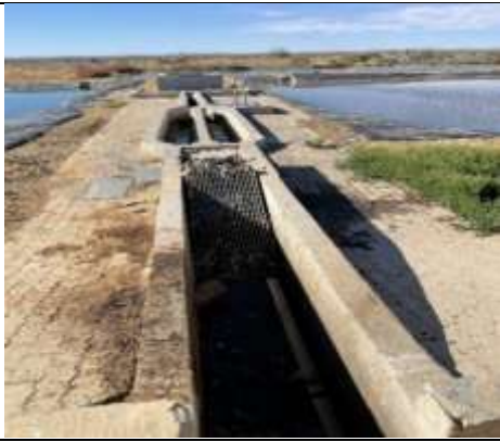
Grit channels installed on site
