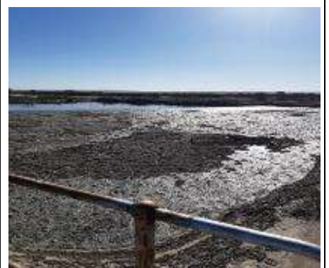
Pond systems are visually overloaded and no sludge removal scheduled
