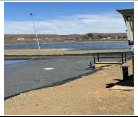
No desludging of anaerobic ponds
