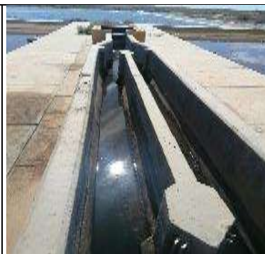
Infrastructure is in place and well maintained
