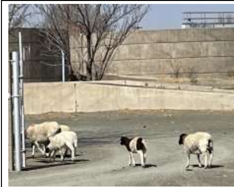
Damaged fence allows for pedestrians and livestock to access the works
