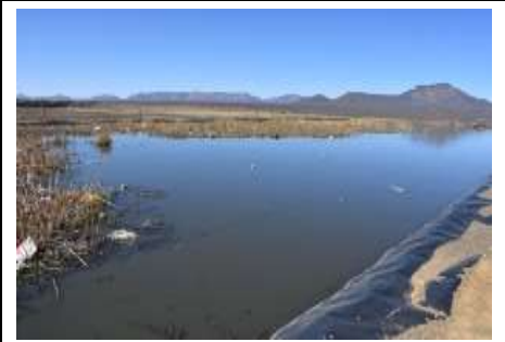
Reedbeds need to be maintained to polish the effluent from the ponds
