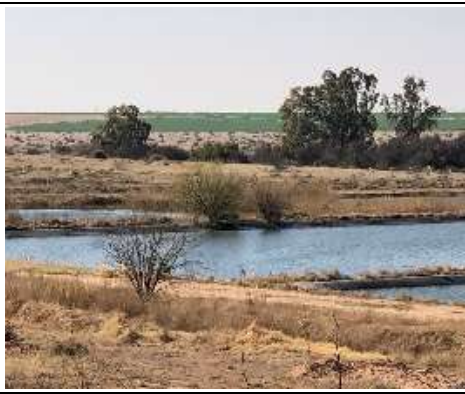
Vegetation (trees and bushes) around ponds may cause damage to dam linings. Must be removed
