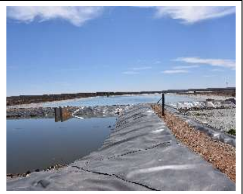
Ponds are adequately lined and structurally sound
