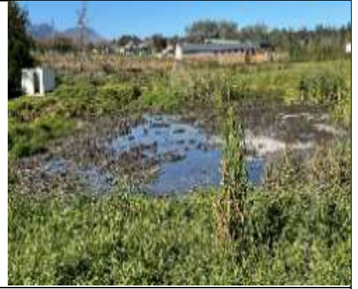
Sludge is treated in unlined sludge ponds. Poor terrain maintenance noted
