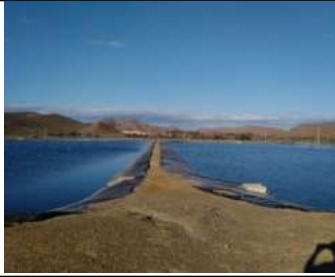
Ponds are lined and in good condition
