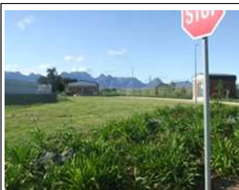
Excellent terrain maintenance, faultless housekeeping of the entire plant – high worker satisfaction and inducive work environment
