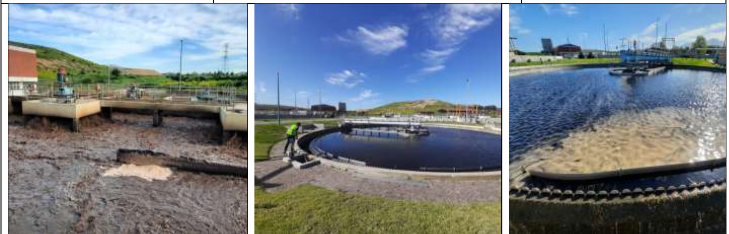
The terrain in very neat, with committed and proud staff, Activated sludge process is well managed and monitored by a top laboratory
