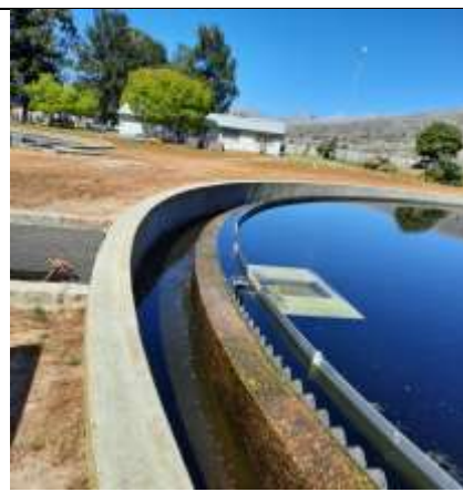
Efficient clarification of effluent resulting in clear overflow and solids clarification with optimised TS content
