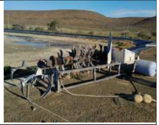
Replacement of floating aerators underway
