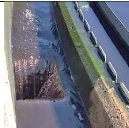
A typical red coloured tint to the final treated industrial water leaving the clarifier on its way to the maturation ponds.
