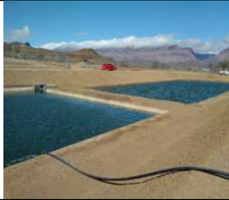
Newly constructed site, ponds are lined, reeds still to be established
