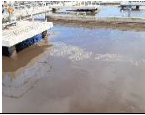
MLSS, DO and sludge age maintained at optimal levels by process controllers
