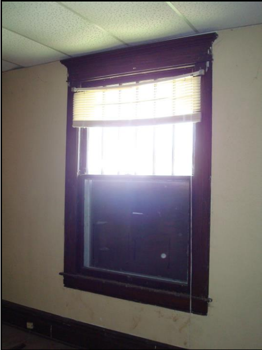
Photo 13. Leaded glass window in living room, first floor interior, facing south
