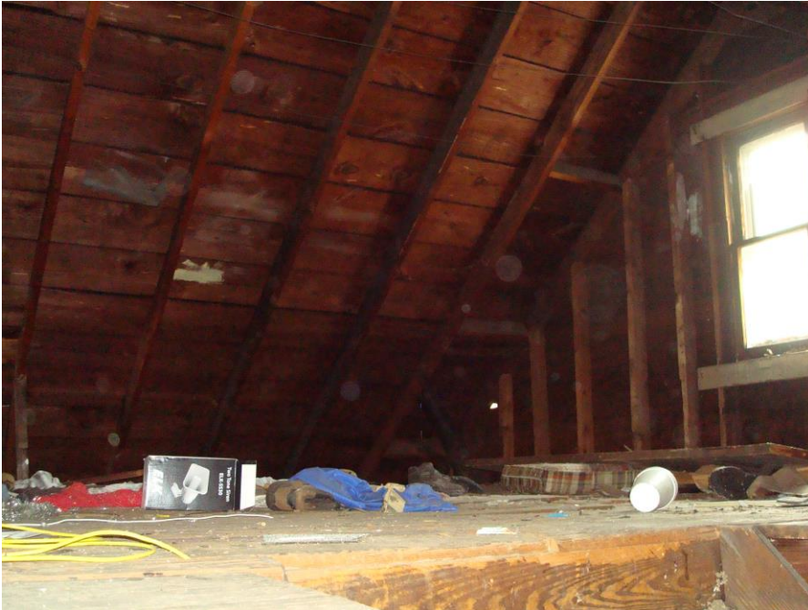
Photo 27. Attic, facing northeast.
