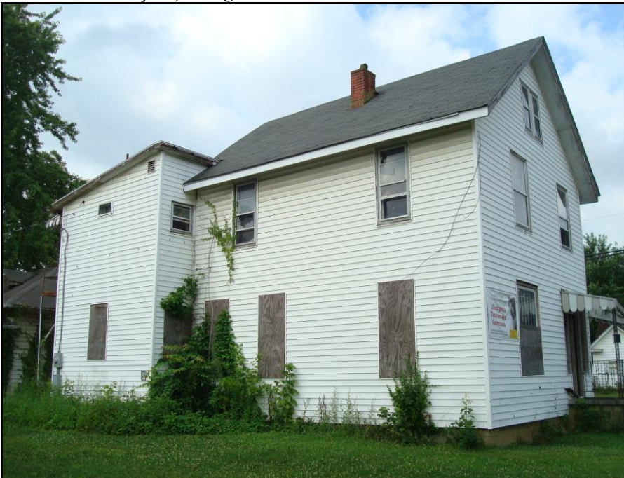
Photo 2. Eastern elevation, facing Southwest of 10 th Avenue.
