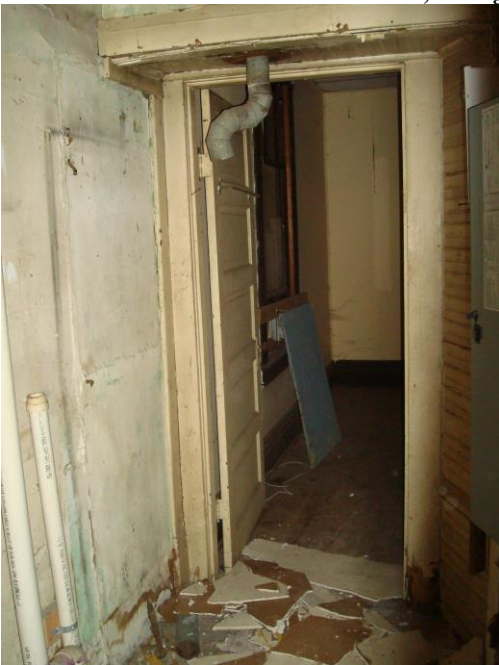
Photo 20: Hallway connecting kitchen and bedroom in first floor addition, facing west from kitchen
