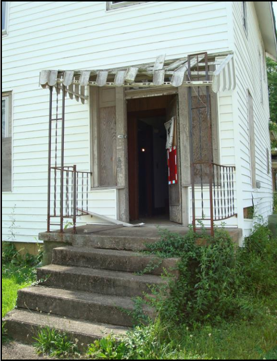
Photo 5. Entryway on front (north) façade, facing south
