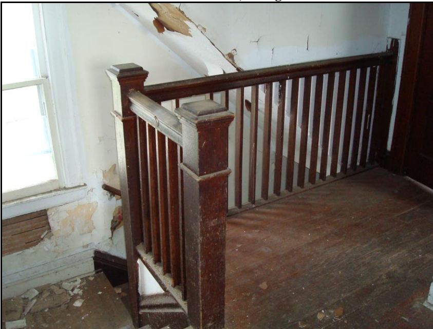
Photo 22. Original staircase balustrade, second floor, facing west
