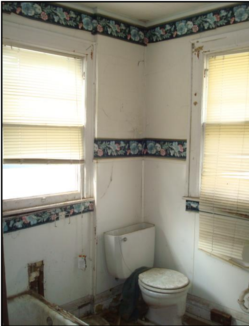
Photo 23. Second Floor bathroom, facing southwest
