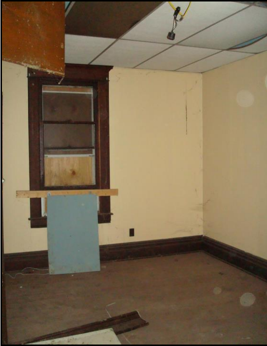
Photo 21. Bedroom in first floor addition, facing south
