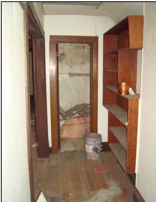
Photo 10. Hallway from entry to bathroom, first floor interior, large built in shelf to west, dining room to east.
