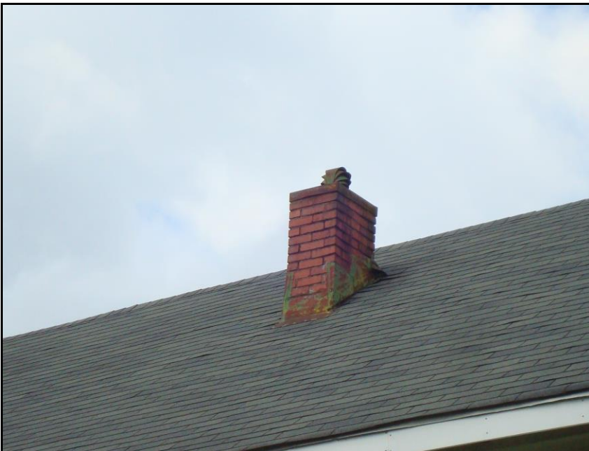
Photo 4. Chimney with cap, eastern of roof, facing west.
