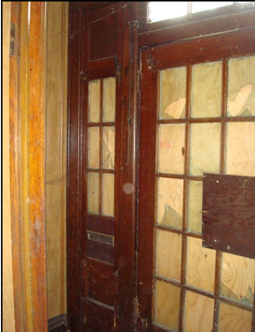
Photo 9. Western side of entry door with sidelight and transom, first floor interior.
