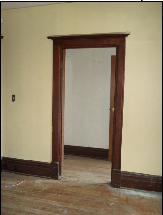
Photo 12: Doorway between living room and entry, first floor interior, facing west.
