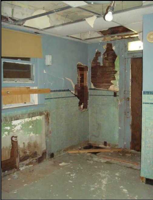
Photo 19. First floor kitchen addition, facing southeast
