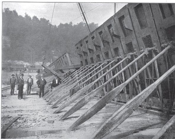
Figure 22. Dam No. 6 on the Ohio River showing wickets and props (Thomas and Watt 1903). The wickets were raised and lowered as needed to adjust upstream water levels.
