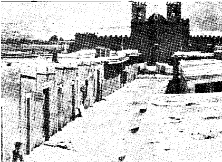
Looking up San Francisco street towards the fifth church of 1806, as first photographed around 1850. Museum of New Mexico.
